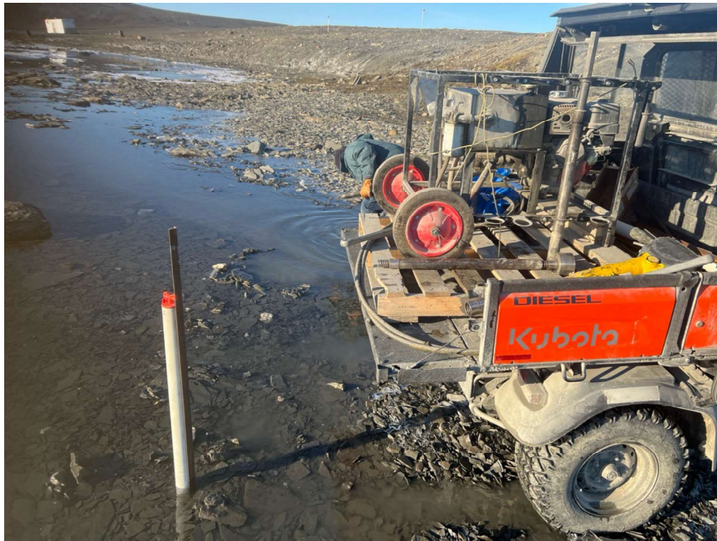
Figure 7: Still well installation at outlet of Upper Dumbell Lake.
