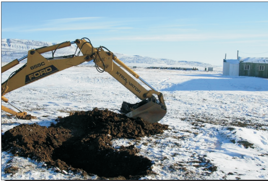
Photo 7 Area 3, DND Barrel Landfill - looking east at excavation test pit.
