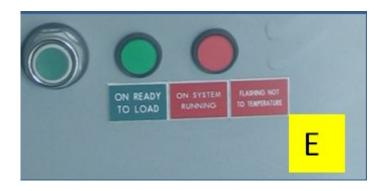
Figure 11 Sub-Section D: Temperature Controllers; E: PLC Indicating Lights and Control Button [CP6 to CP10 in Table 7]
