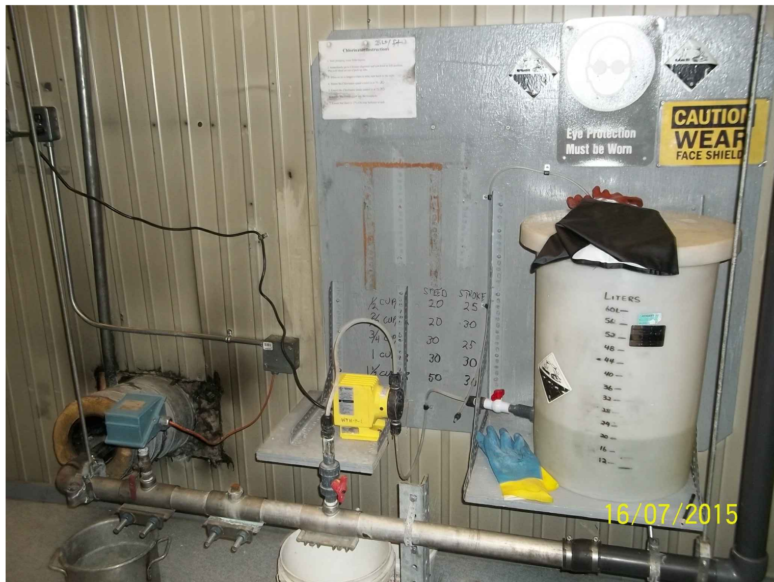
2 | EXISTING CHLORINATION SYSTEM FOR DEMOLITION
