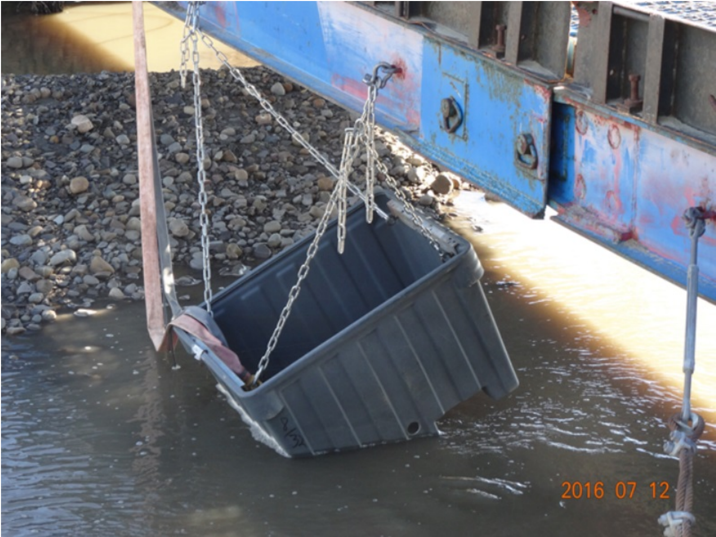
Figure 3 Intake- Submersible pump located within the suspended box unit
