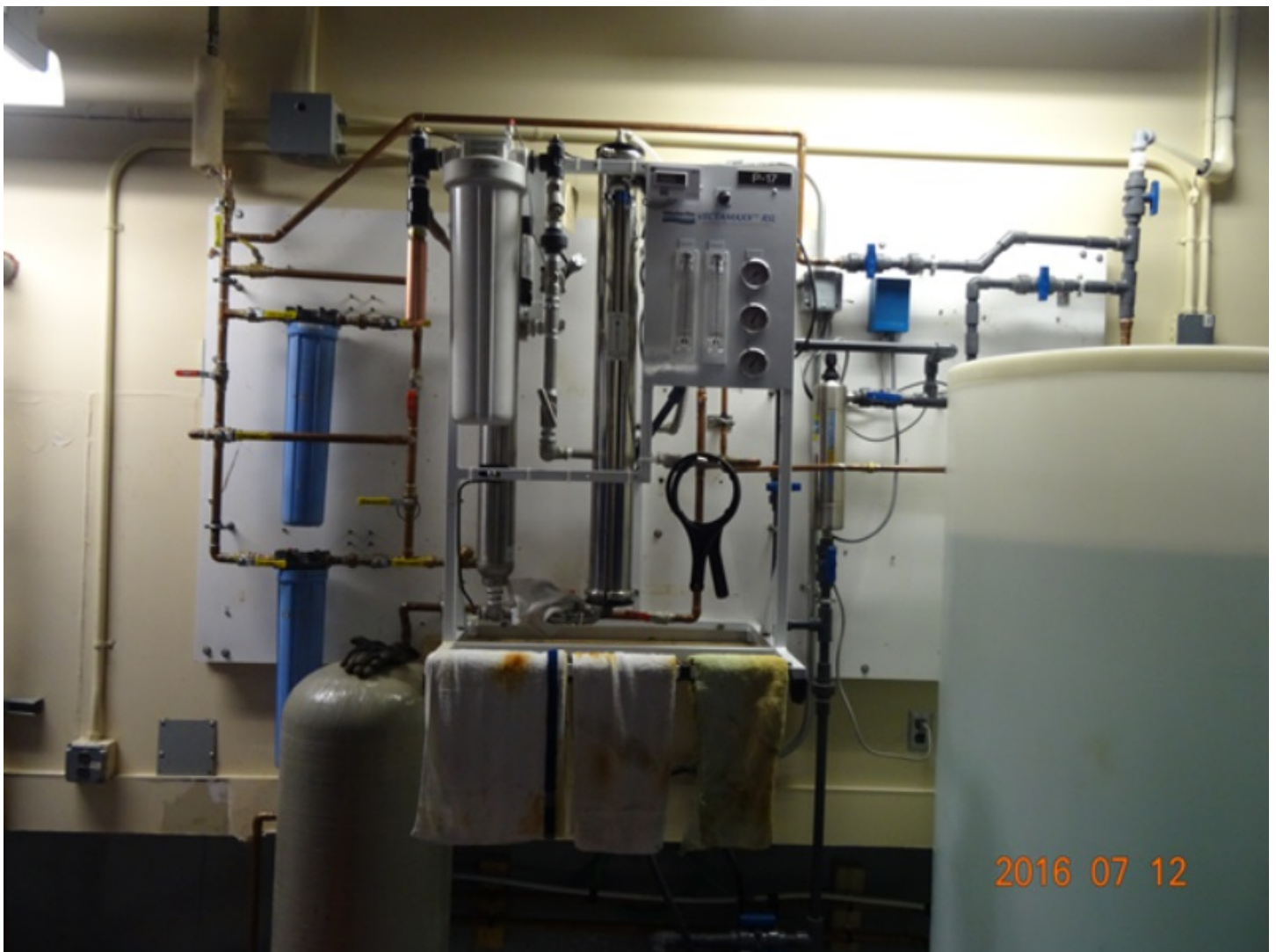
Figure 7 Water treatment including reverse osmosis machine
