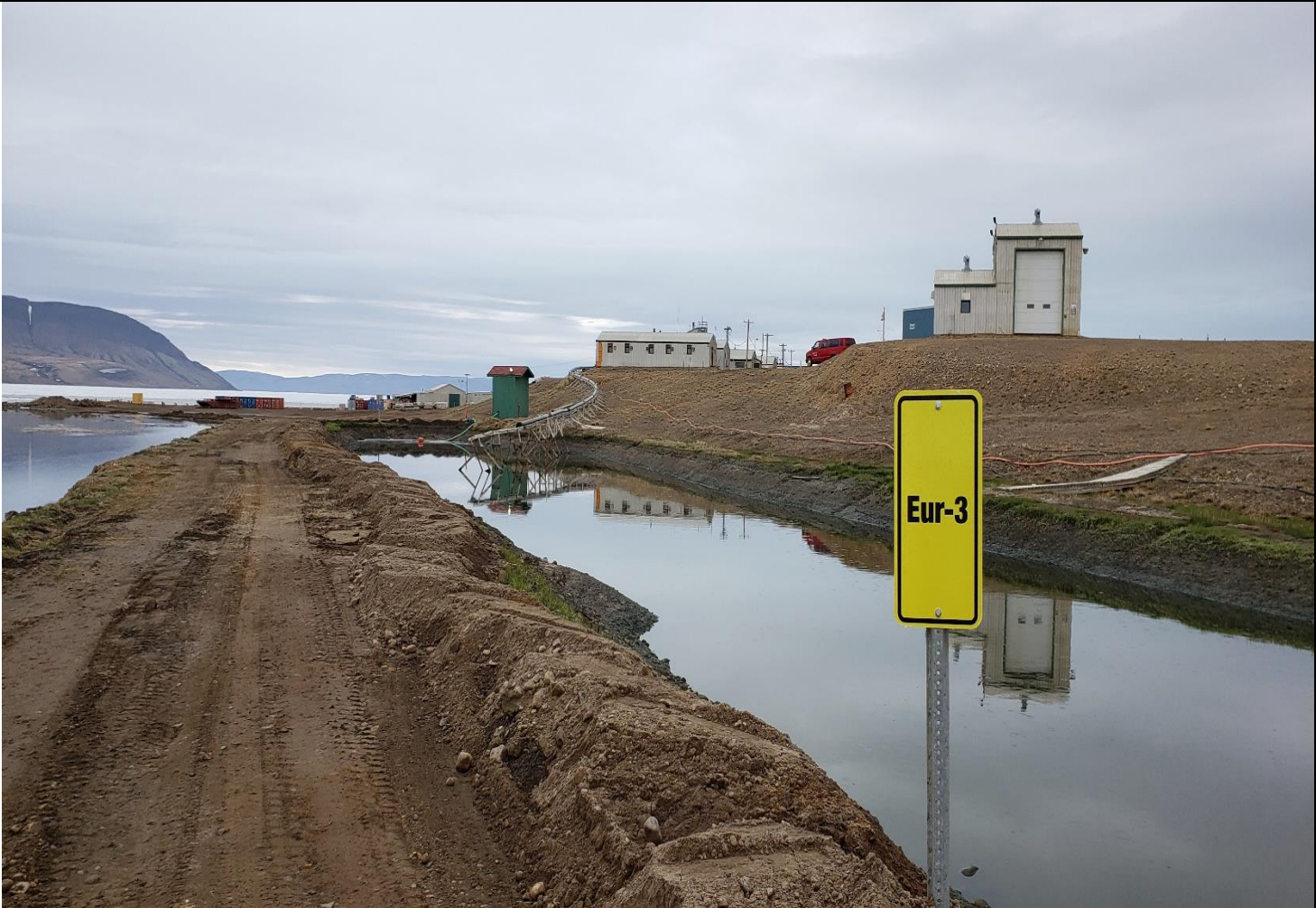
Description: Eur-3 monitoring station. sewage lagoon fills up by pipe, and trucks.
