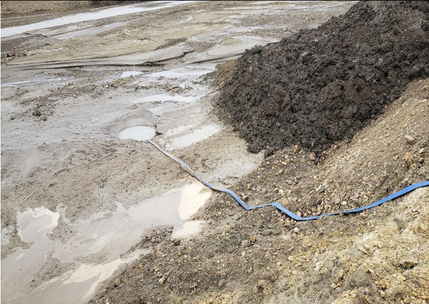
Description: Wet loam observed. install silt fencing to mitigate the potential for sedimentation in the river. River at low mark in the top right background. Sedimentation observed along the base of the newly laid reservoir walls, within the high mark of the river. No direct observation of sedimentation into the river.
