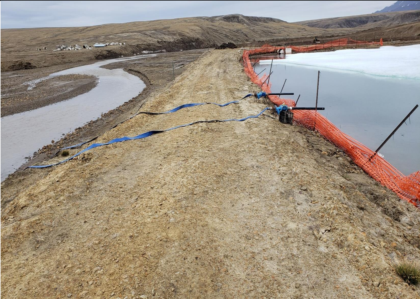
Description: Water reservoir recharge location for 2022. Some parts of the reservoir was less than 1 metre freeboard. Water meters on pump.
