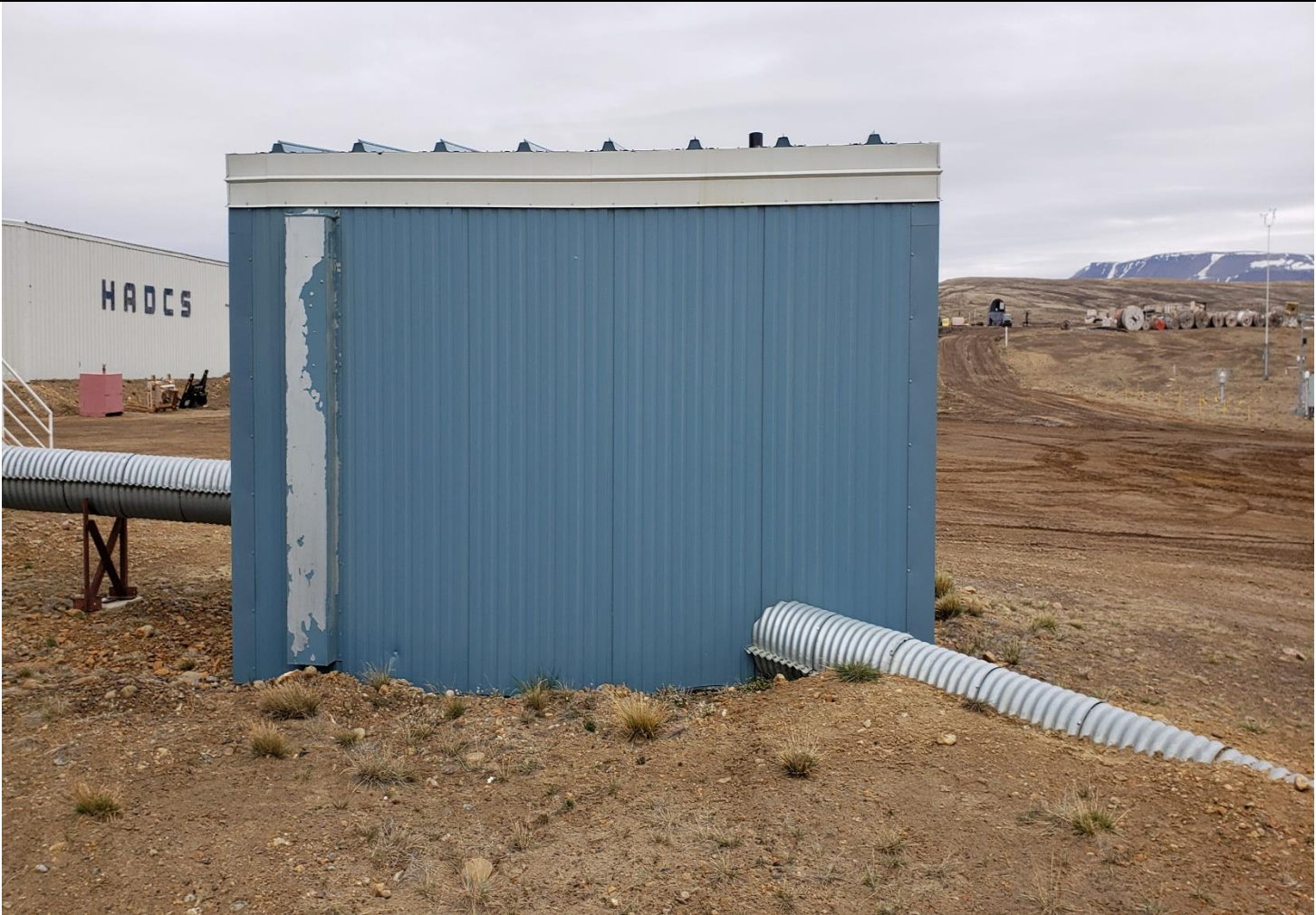
Description: liquid waste, and solid was exit the accommodations, and office building into the sump tank building.
