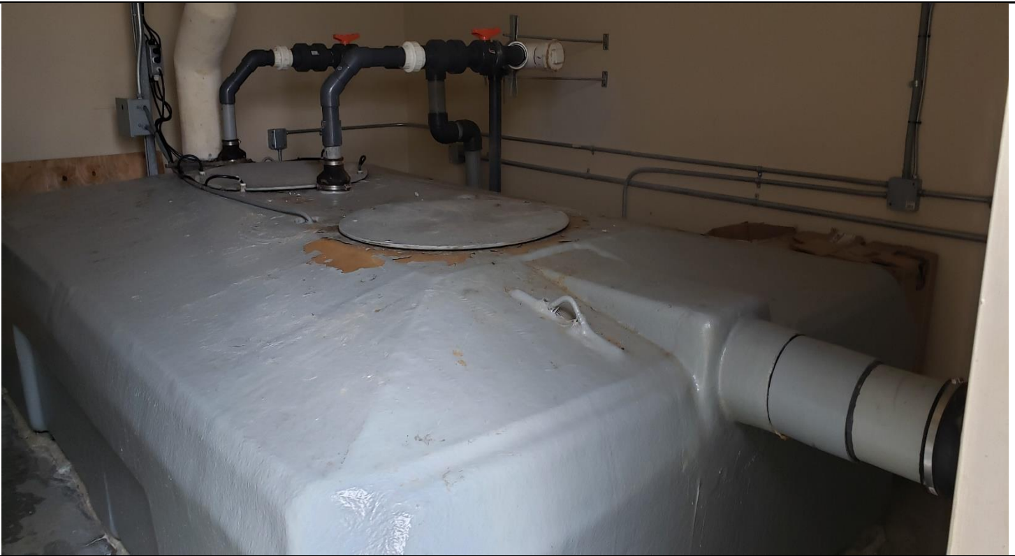
Description: Sump tank, before being discharged to the sewage lagoon.
