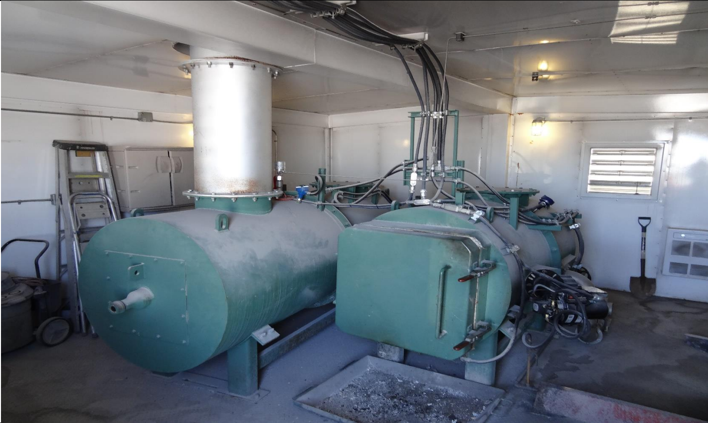
Description: Forced Air Incinerator on site. Photo submitted by ECCC. All waste ash appears to be contained within building.
