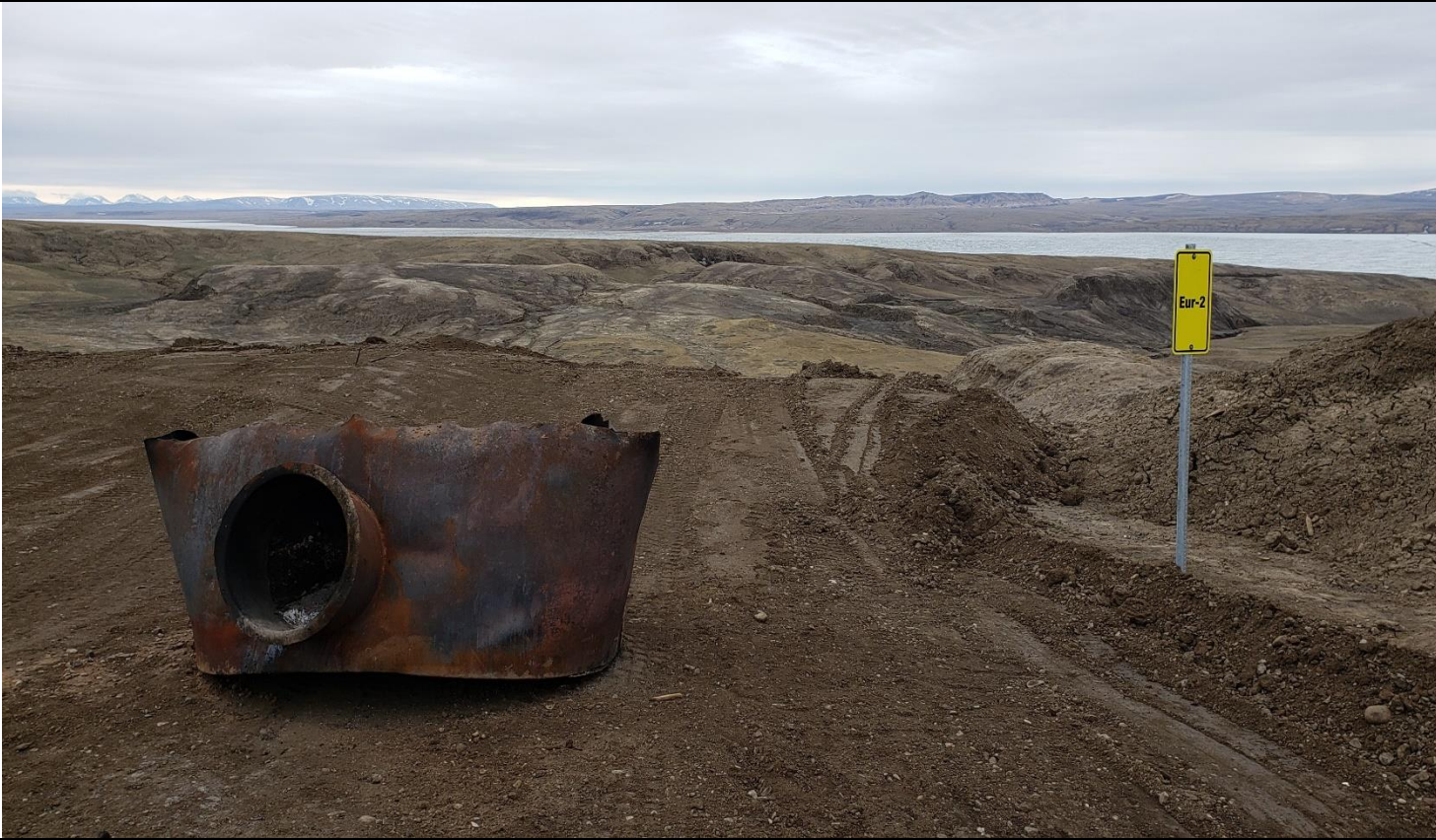
Description: landfill, burn and cap. Solid waste is pushed off the left hand side of the sign, and capped with gravel. EUR-2 is observed as the monitoring station.
