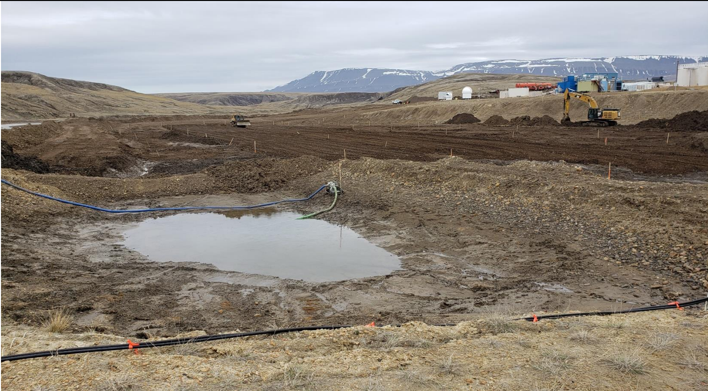
Description: At the time of the inspection, work was being done to expand the capacity of the water reservoir.
