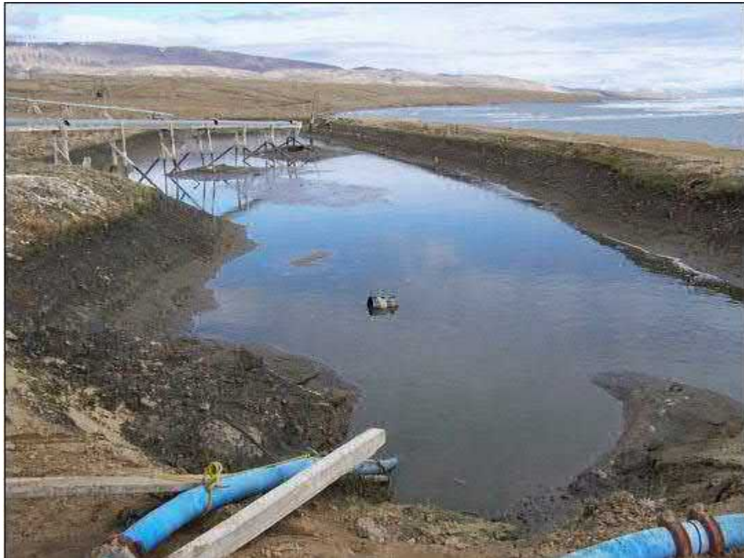
Figure 2. Wastewater Sewage Lagoon at Eureka HAWS
