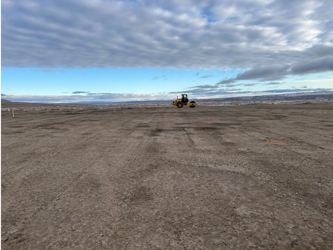
Photo: Compacting south-west berm.
