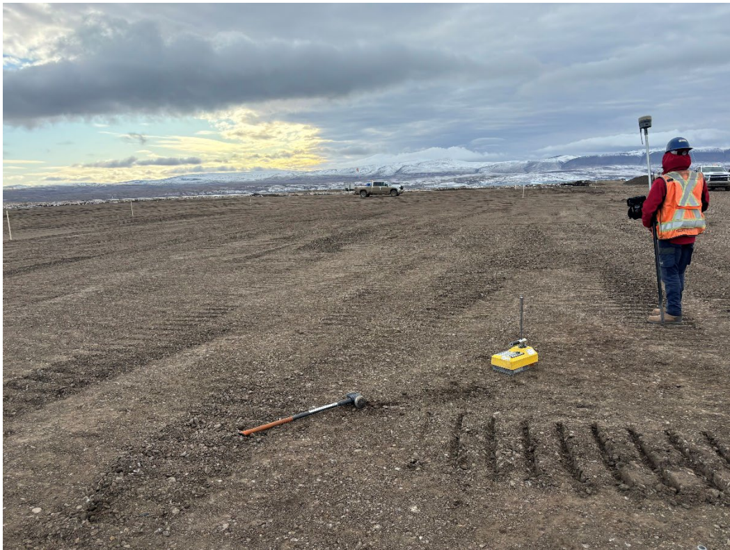
Photo: Failed compaction test on south half of STF.
