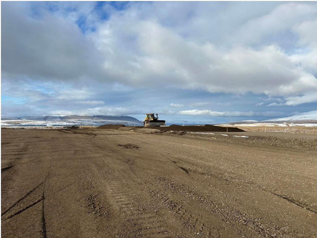
Photo: Dozer pushing material for 250mm lift on north-west berm.
