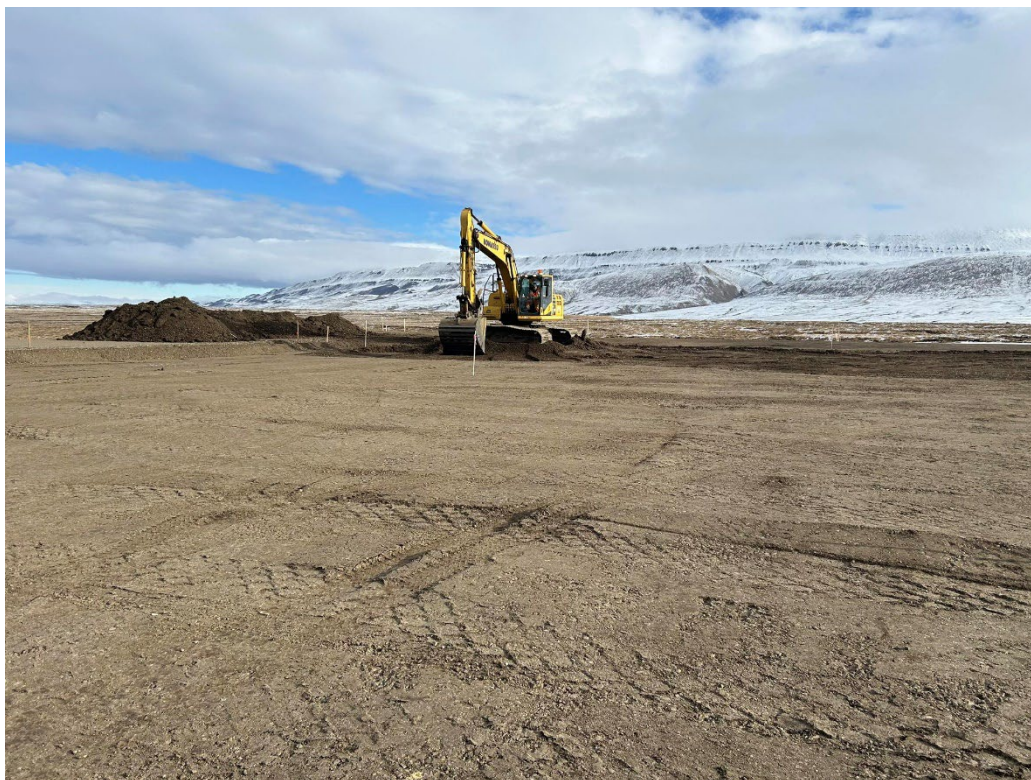
Photo: Excavator trimming down high area in north-east corner.
