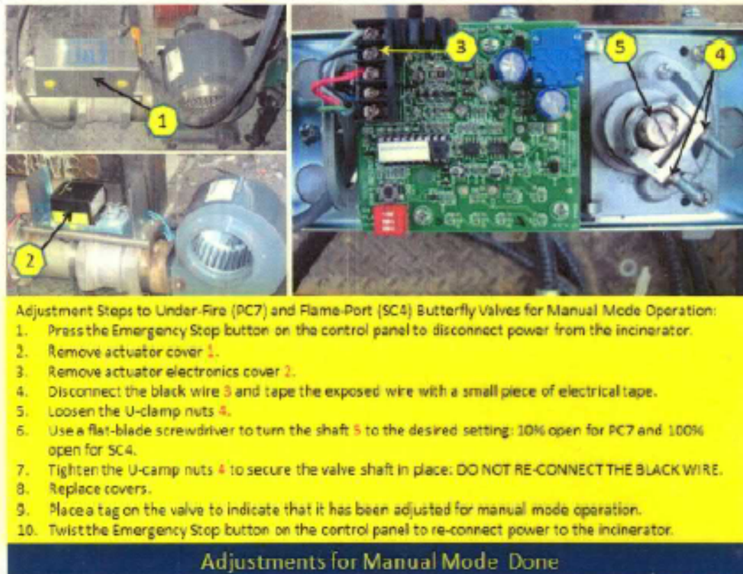
Figure 17 Butterfly Valve Adjustment for Manual Mode Operation
