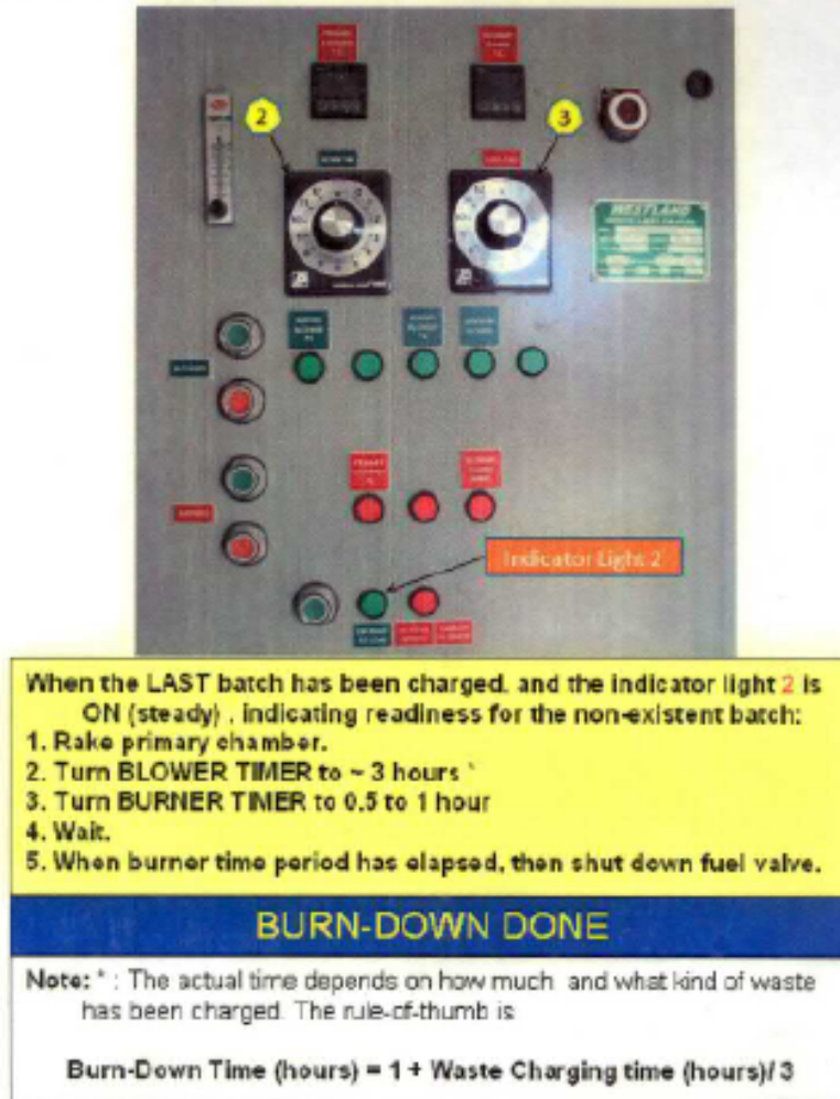
Figure 15 Procedure for Burn Down
