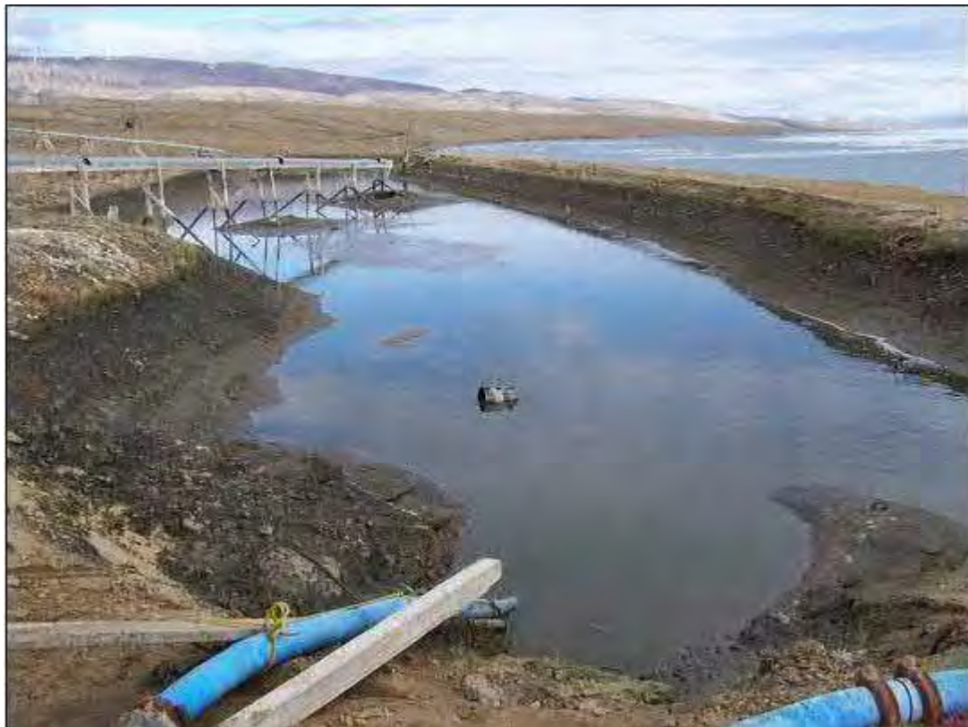
Figure 2. Wastewater Sewage Lagoon at Eureka HAWS
