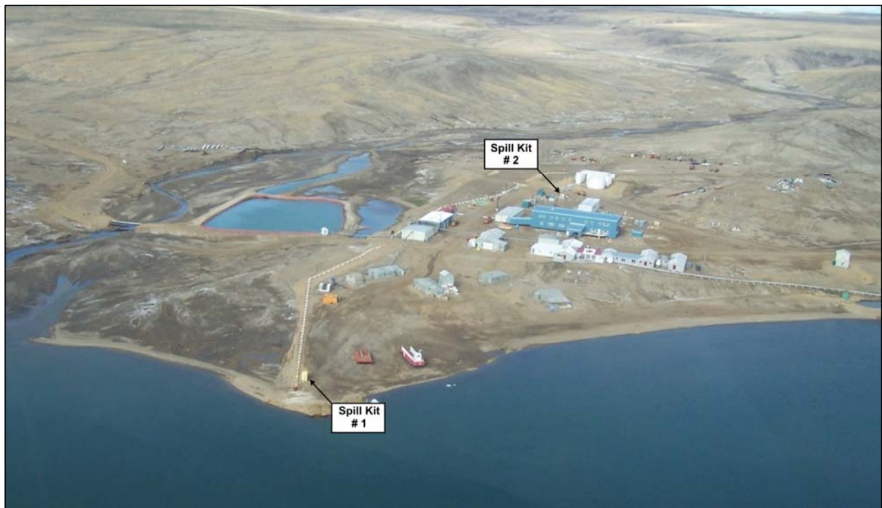
Figure 3. Eureka HAWS showing locations of the two on-site spill kits.
