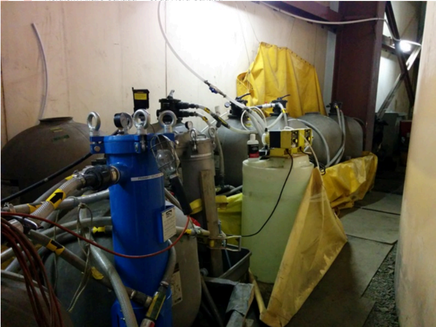
Figure 23 Hydrogen Peroxide infusion and carbon filtration systems in place on site A.Wingardener
