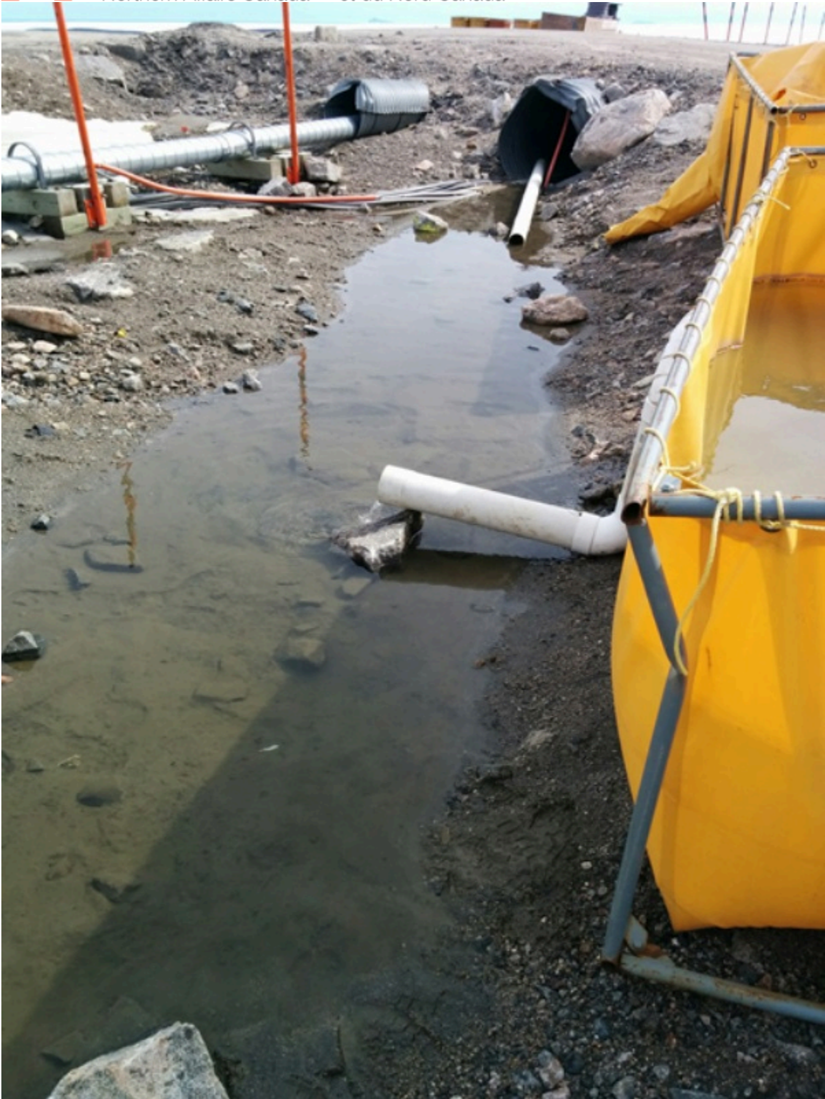
Figure 19 Direct discharge of treated hydrocarbon impacted water
