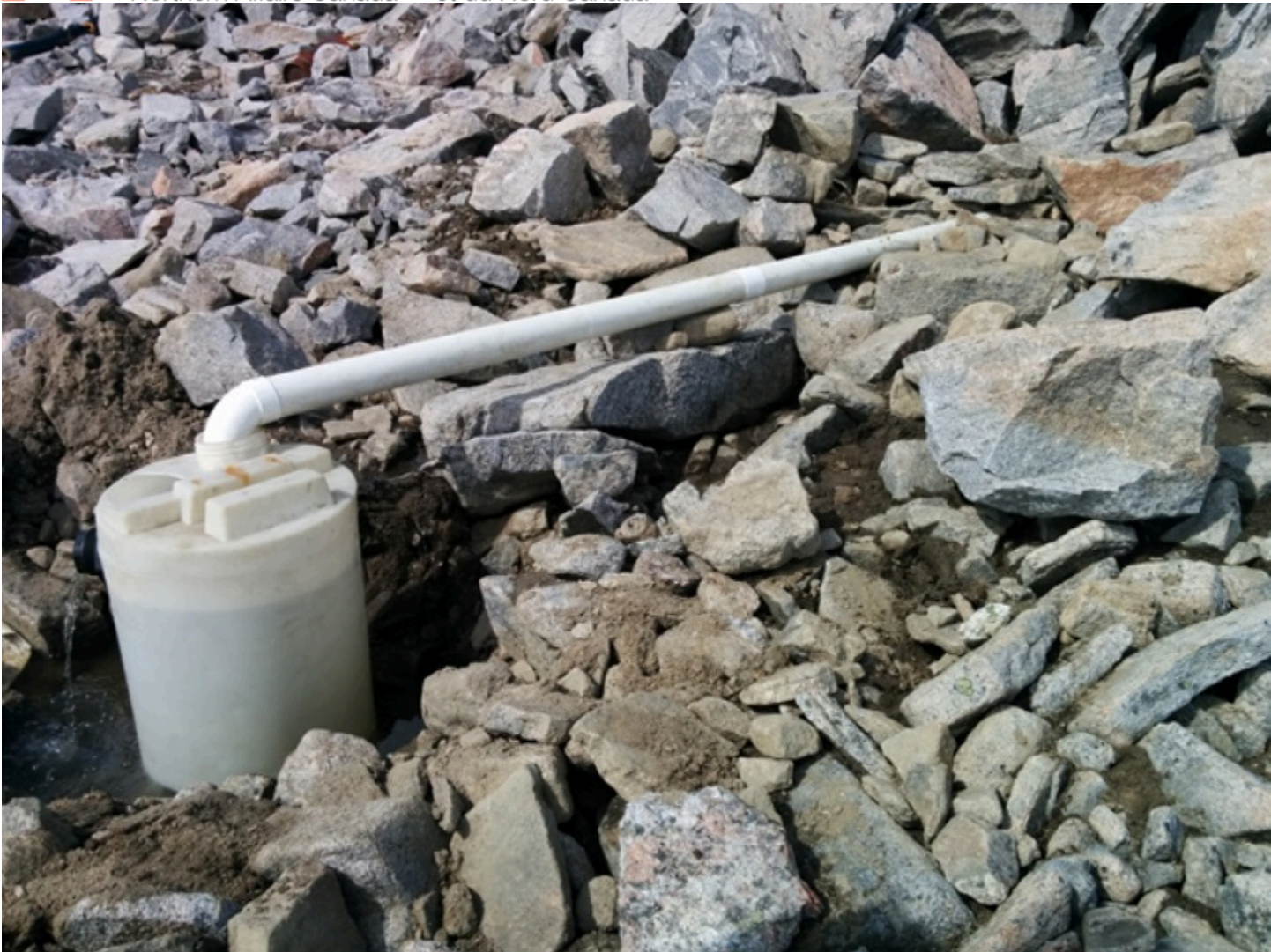
Figure 26 Oil Trap installed on south side to catch surface flow A.Winegardener
