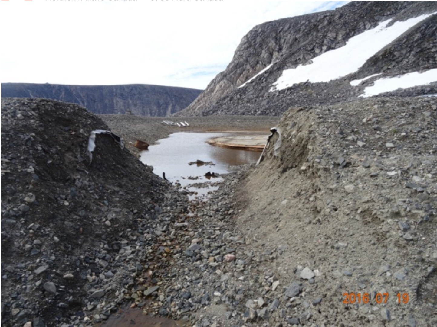
Figure 4 Legacy Beach tank removal project - Berm wall breach to remove water (2015)
