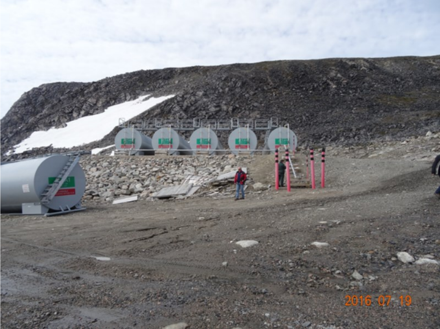
Figure 1 Beach tank farm. New tanks (5) Five in-service and two awaiting installation
