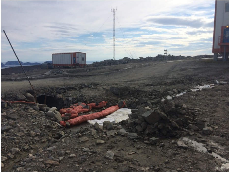
Photo 1. North of TSM looking NE, booms and pads placed downgradient in evidence. August 8, 2015.
