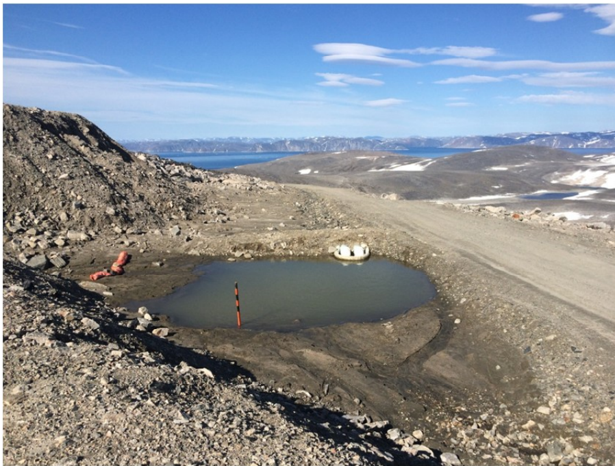
Photo 4. Stormwater pond with intact underflow dam north of TSM. August 8, 2015.
