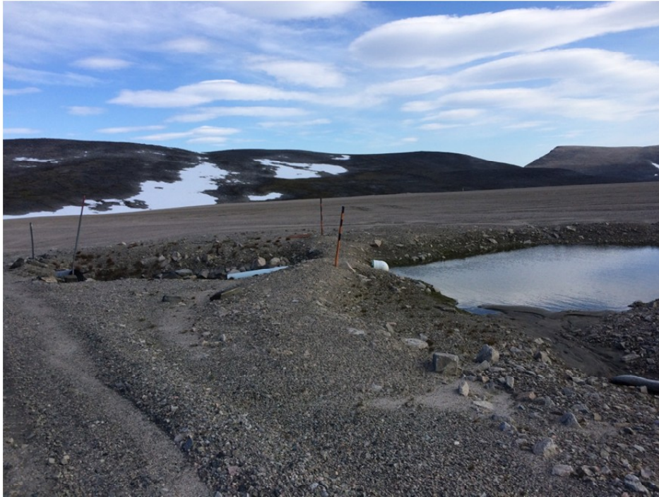
Photo 7. Stormwater pond and underflow dam at middle site. August 8, 2015.
