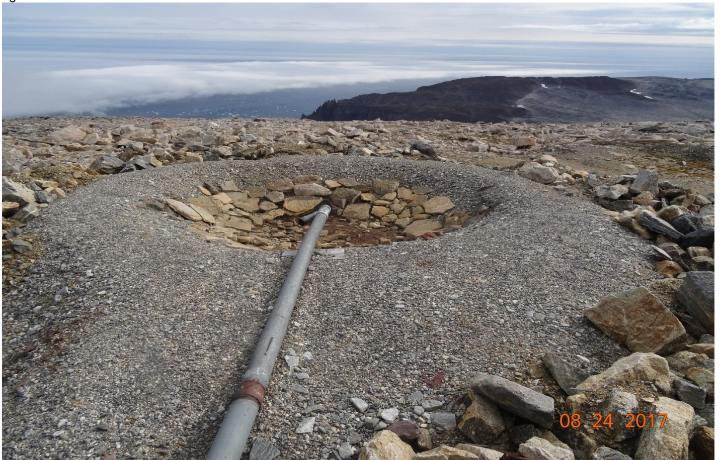
Figure 2: Effluent outfall.
