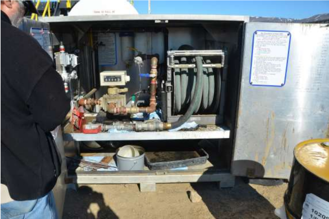
Figure 1- DND North Apron Fuel Dispensing Pump Container.
