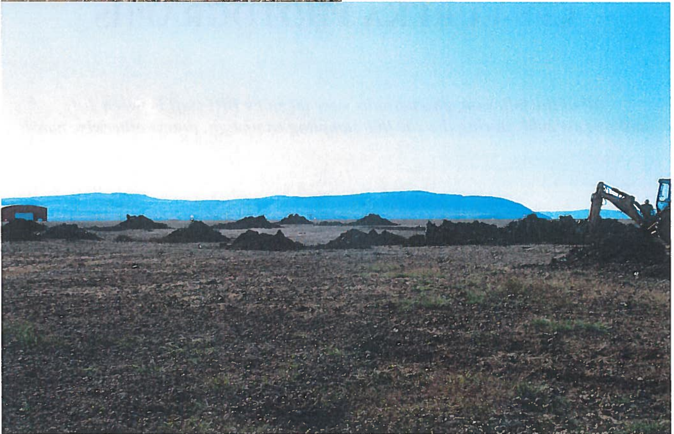
Photograph 16. (North Airstrip Apron, S-10527) Delineated area located south of the 4 tanks.
