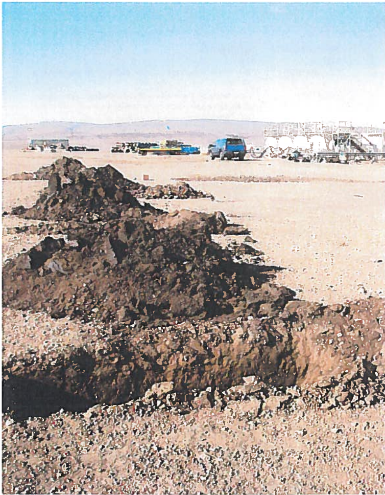
Photograph 17. (North Airstrip Apron, S-10527) Another view of trenches delineating the east edge of the contaminated area.
