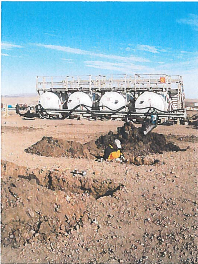
Photograph 15. (North Airstrip Apron, S-10527) Trenches dug in front of the refuelling tanks.
