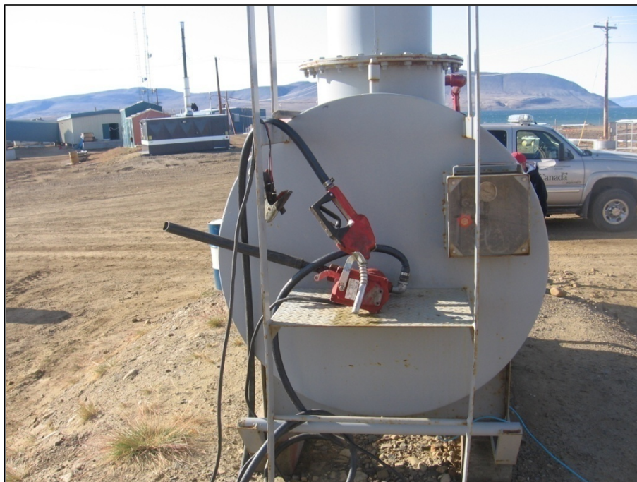
Photo 10: Gasoline Dispensing Tank Product Transfer Area
