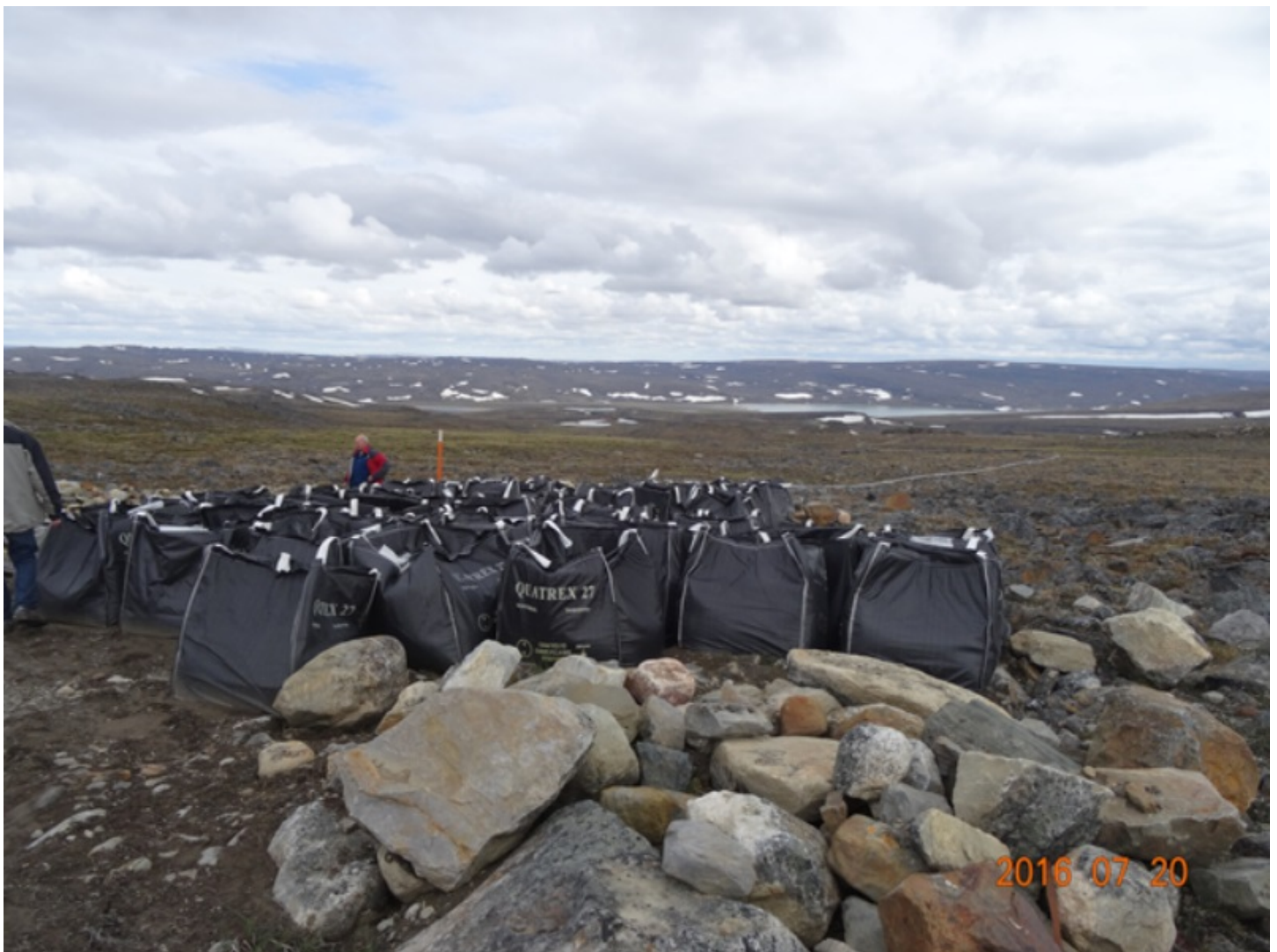
Figure 14 2009-341 - Quatrex bags of PHC soils on pipeline
