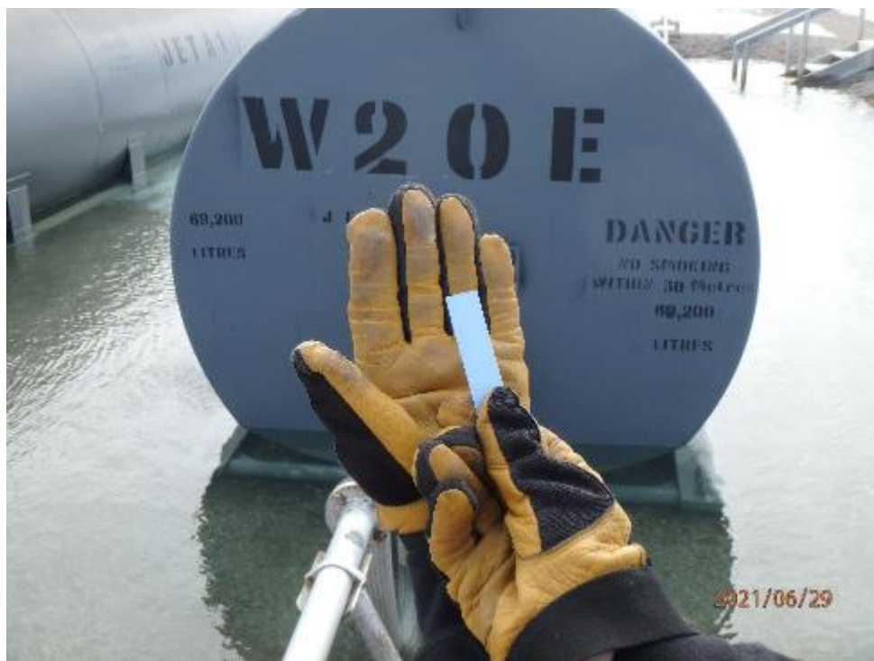
Photo E 6: Hydrocarbon test strips used in berm of tank W20E &amp; W20D (29-Jun-2021)
