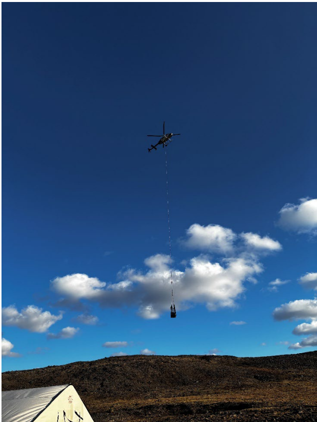
Photo 4 - Helicopter Slinging Materials to Temporary Campsite
