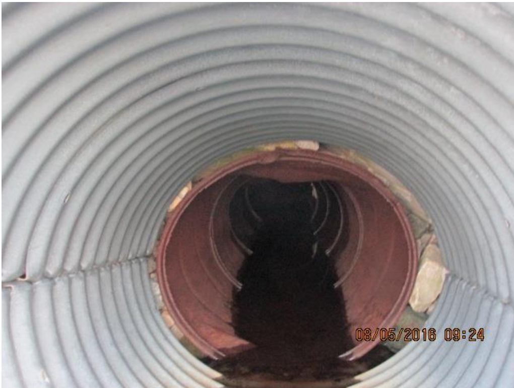
Figure 5: Example on condition of culvert to be replaced in "Area #2"
