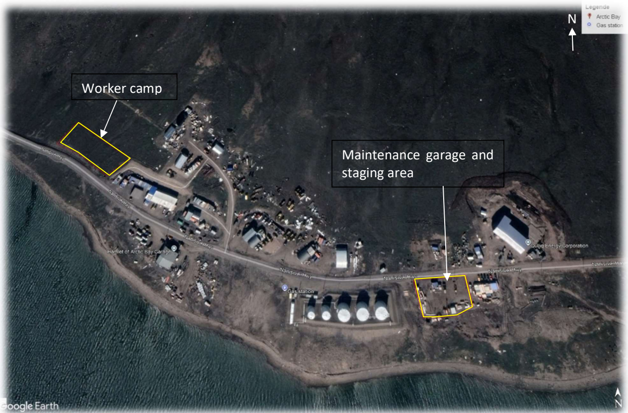
Figure 3.1: Worker camp, maintenance garage and staging area location
