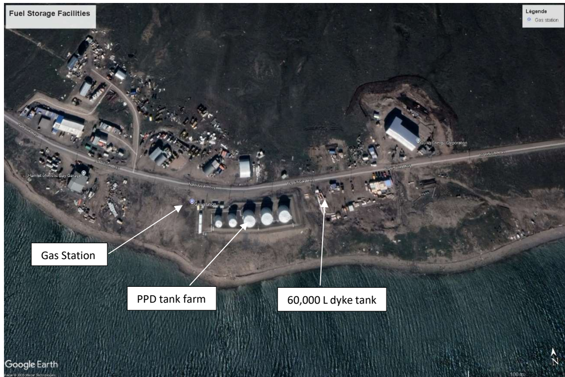
Figure 3.1: Fuel storage in the industrial area
