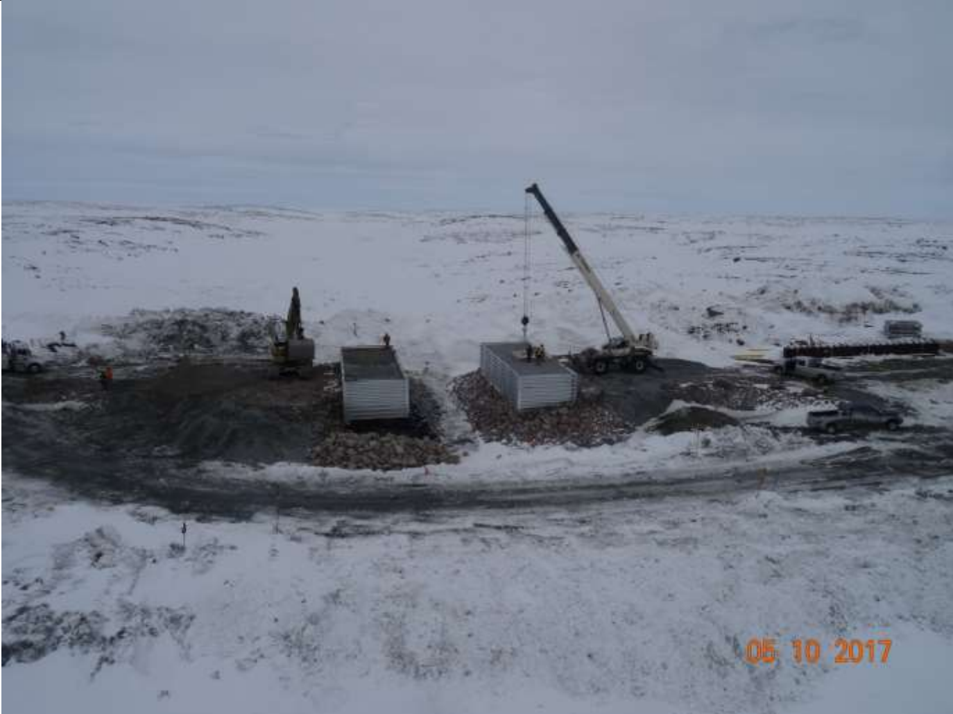
Description: Bridge 32.3KM installation of abutments
