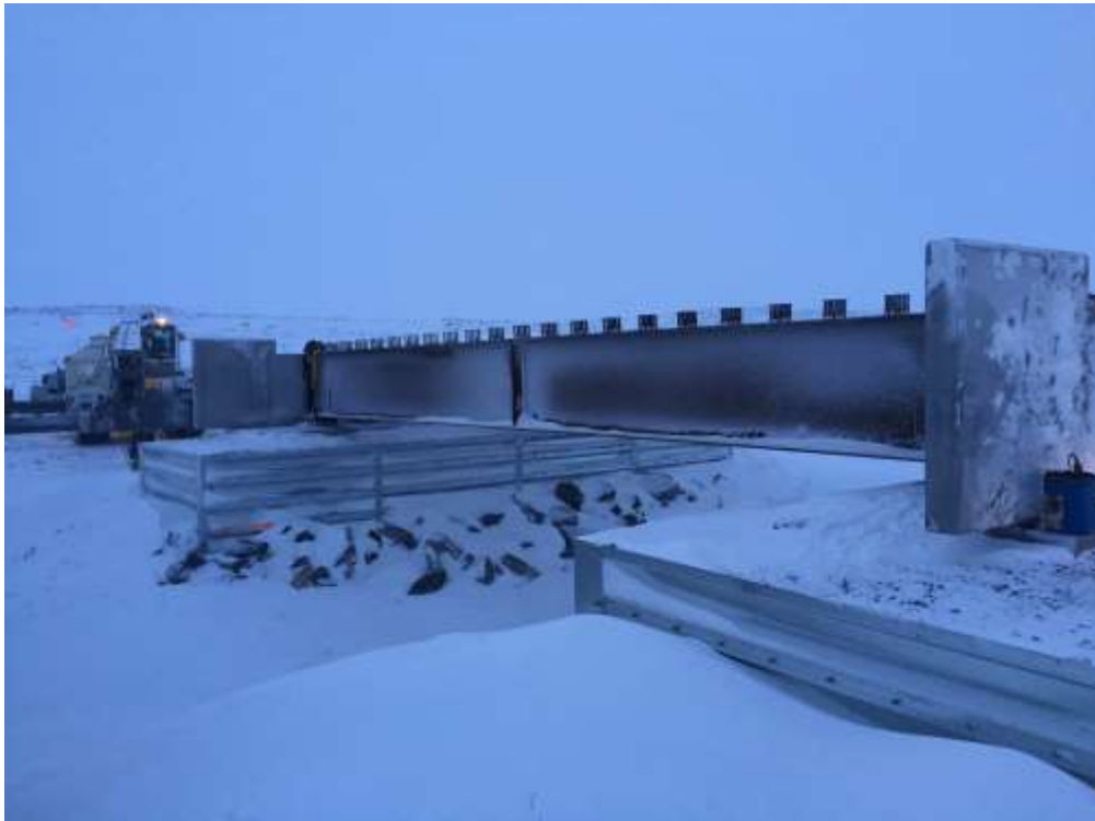
Photo 2: Bridge at KM 10.7 during construction (2016)
