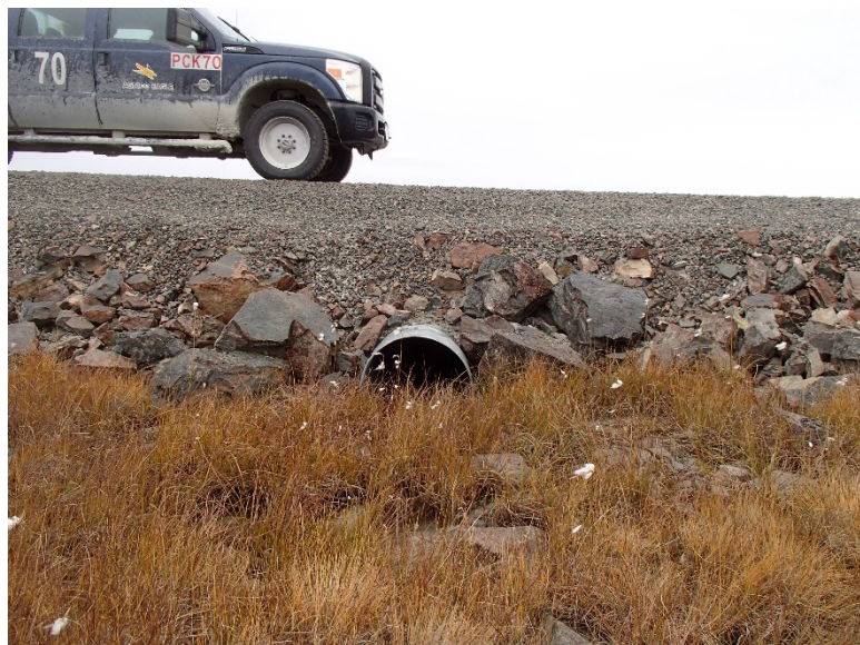
Photograph D1-17: R-03 km 10+580
