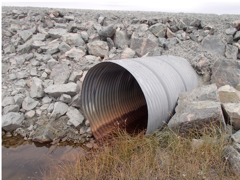
Photograph D1-42: R-07 km 25+900
