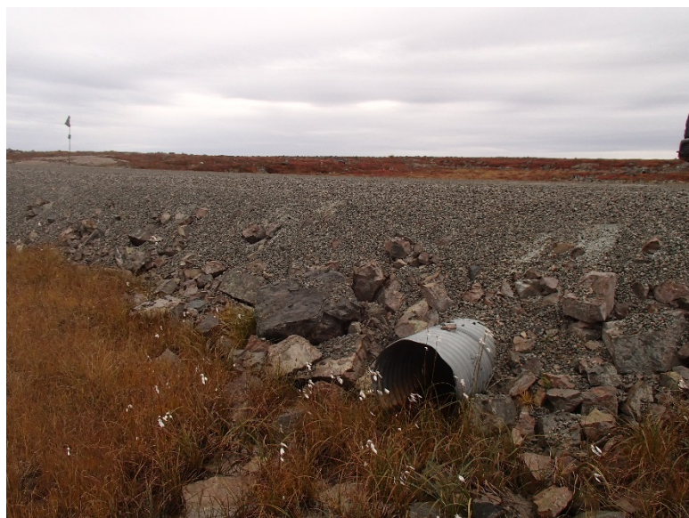
Photograph D1-18: R-03 km 10+580
