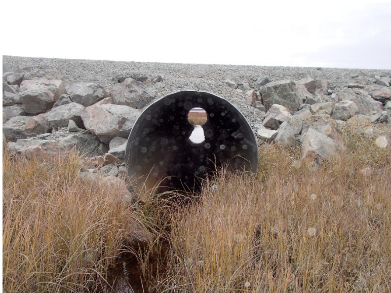
Photograph D1-41: R-07 km 25+900
