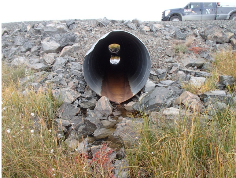
Photograph D1-20: R-04 km 12+050
