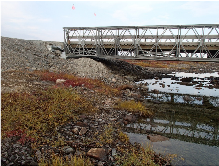
Photograph D2-19 Bridges 6 – R15 km 69+200
