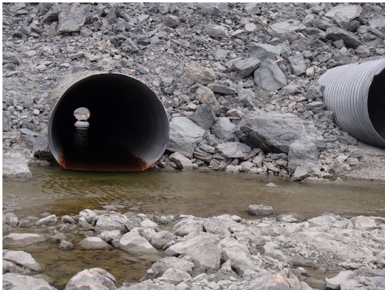
Photograph H1-3 Vault Road Culverts
