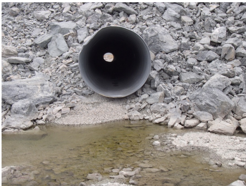
Photograph H1-4 Vault Road Culverts
