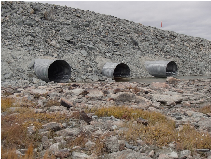
Photograph H1-1 Vault Road Culverts
