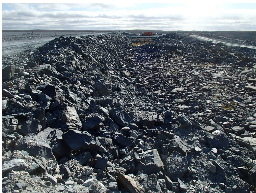
Photograph A3-13 Bay Goose Dike
