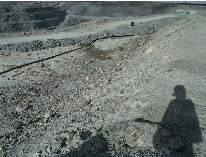
Photograph A3-6 Bay Goose Dike
