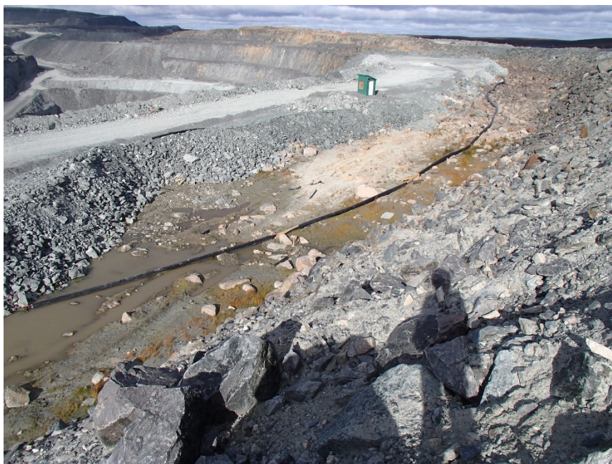
Photograph A3-4 Bay Goose Dike
