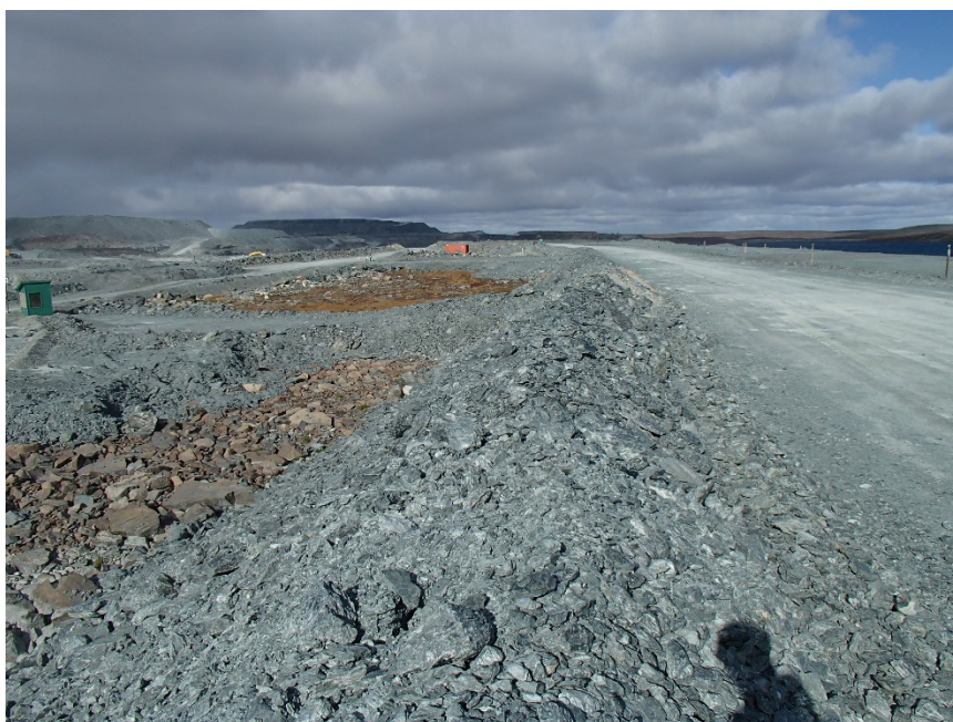
Photograph A3-16 Bay Goose Dike
