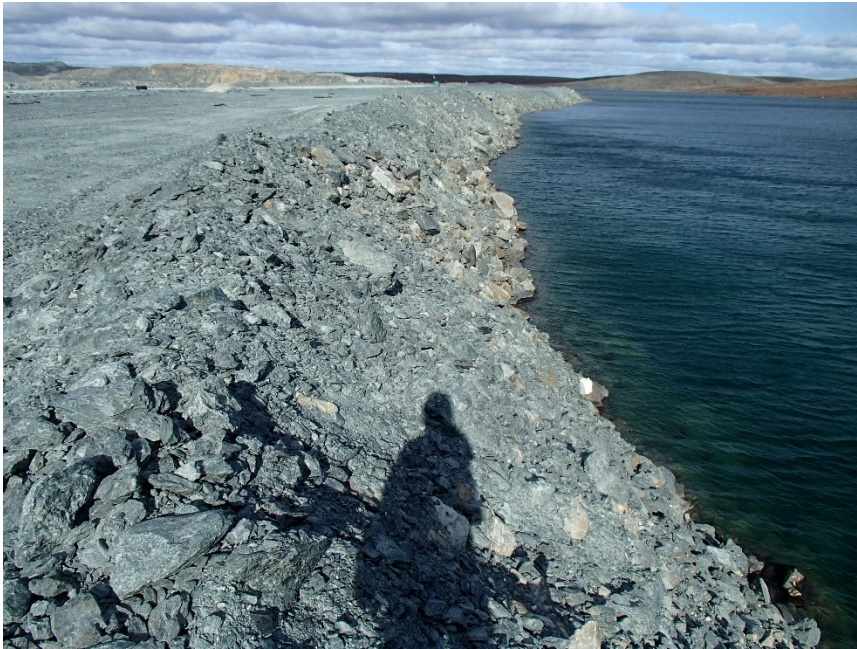
Photograph A3-7 Bay Goose Dike
