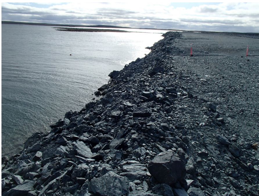
Photograph A3-14 Bay Goose Dike
