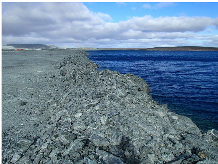
Photograph A3-15 Bay Goose Dike
