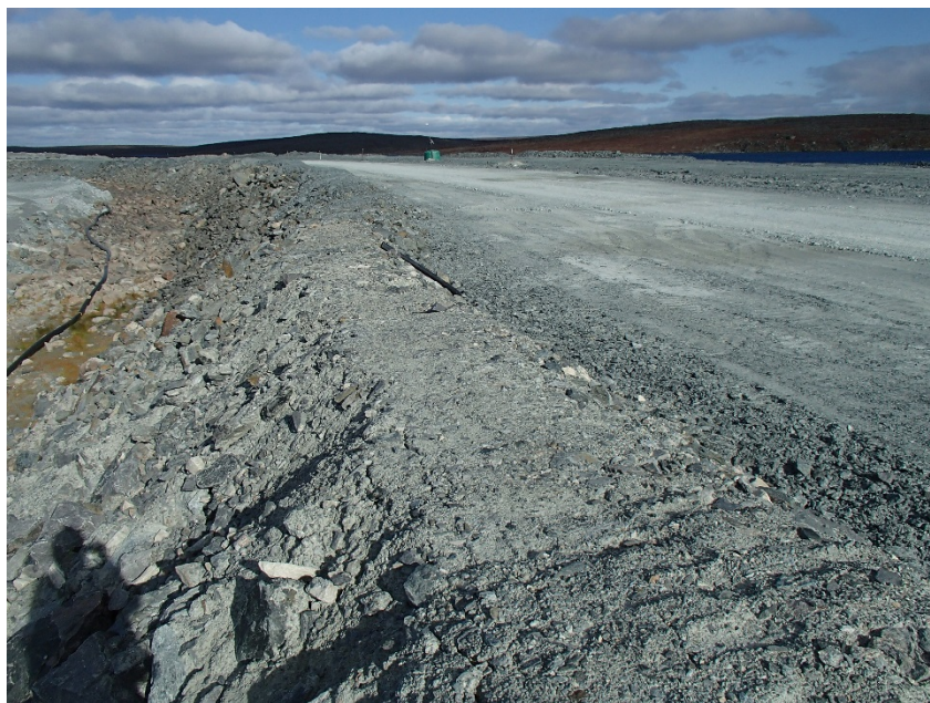
Photograph A3-3 Bay Goose Dike
