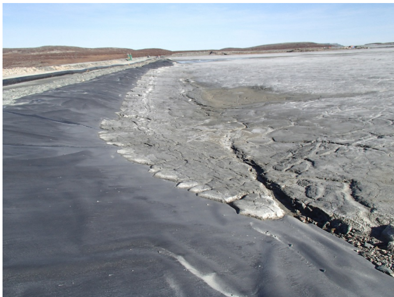
Photograph B2-8 Saddle Dam 1
