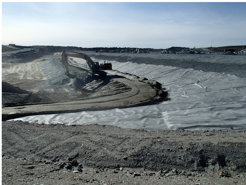
Photograph B5-1 Saddle Dam 3
