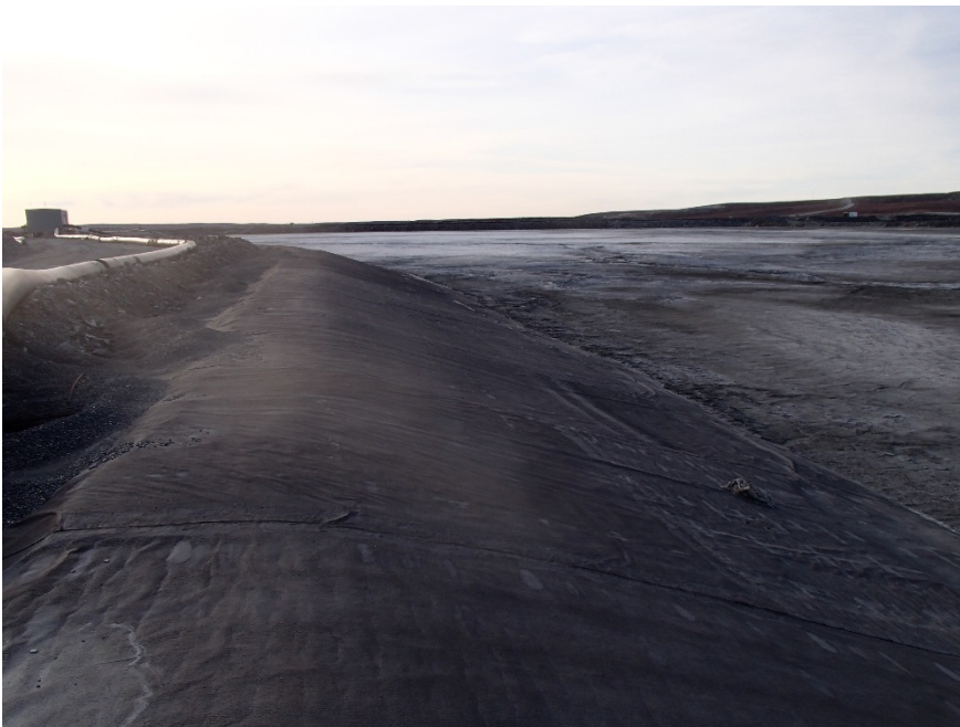
Photograph B7-6 Stormwater Dike
