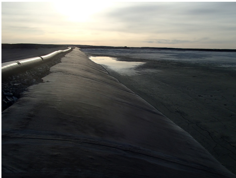
Photograph B4-1 Stormwater Dike
