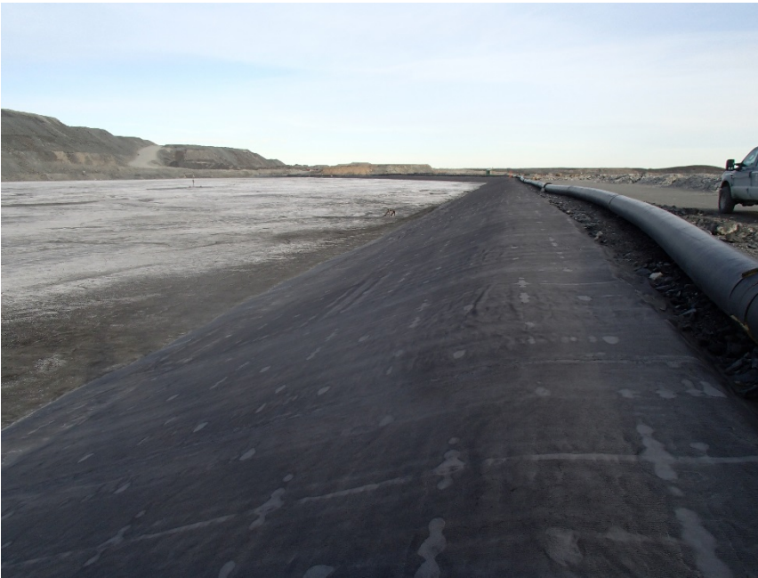
Photograph B7-5 Stormwater Dike
