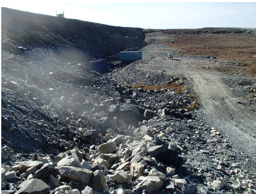
Photograph B2-2 Saddle Dam 1
