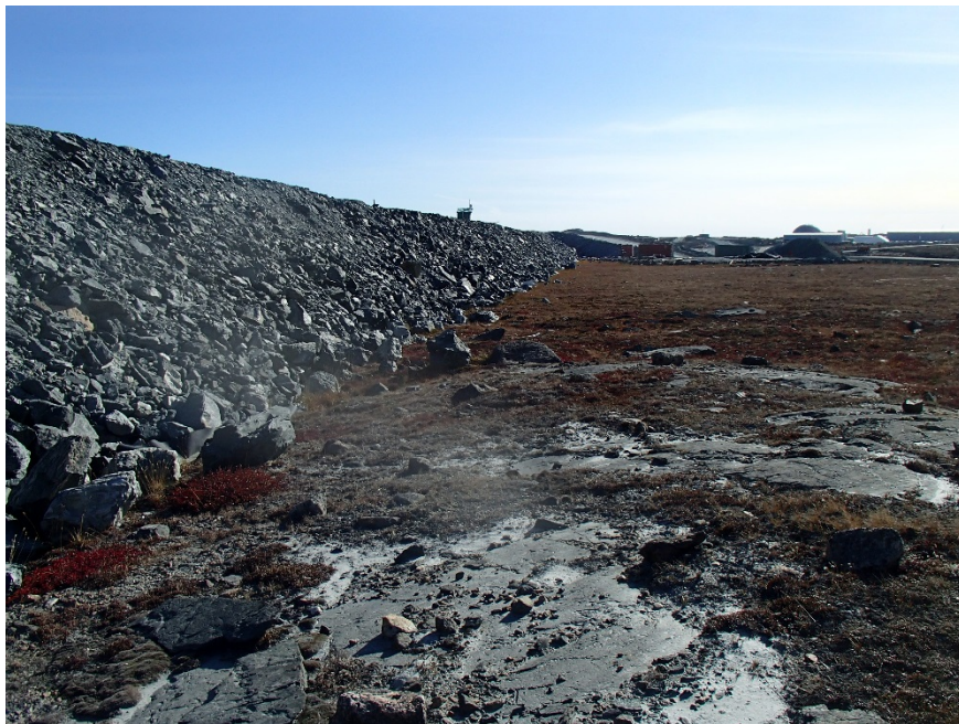
Photograph B3-5 Saddle Dam 2
