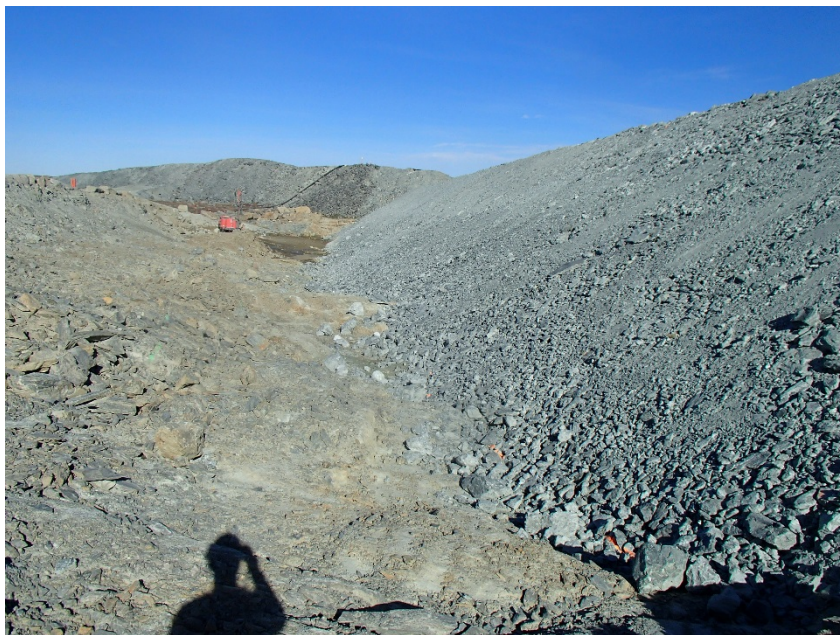
Photograph B5-2 Saddle Dam 3
