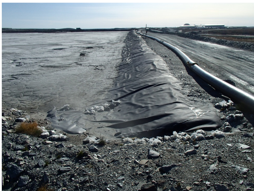
Photograph B3-1 Saddle Dam 2
