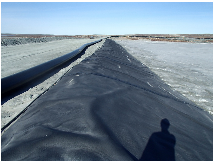
Photograph B3-3 Saddle Dam 2
