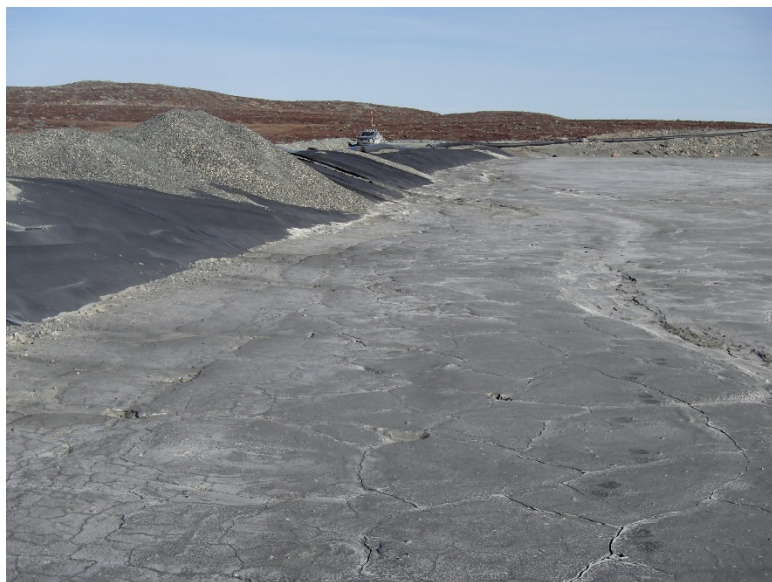
Photograph B2-7 Saddle Dam 1
