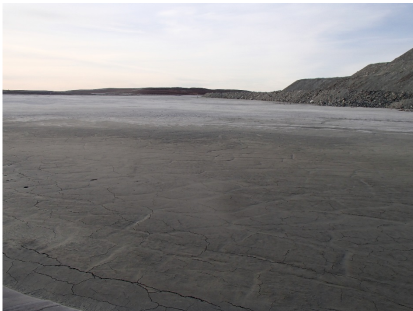
Photograph B4-2 Stormwater Dike
