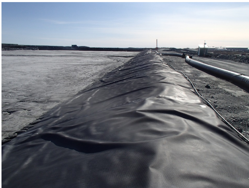
Photograph B3-2 Saddle Dam 2
