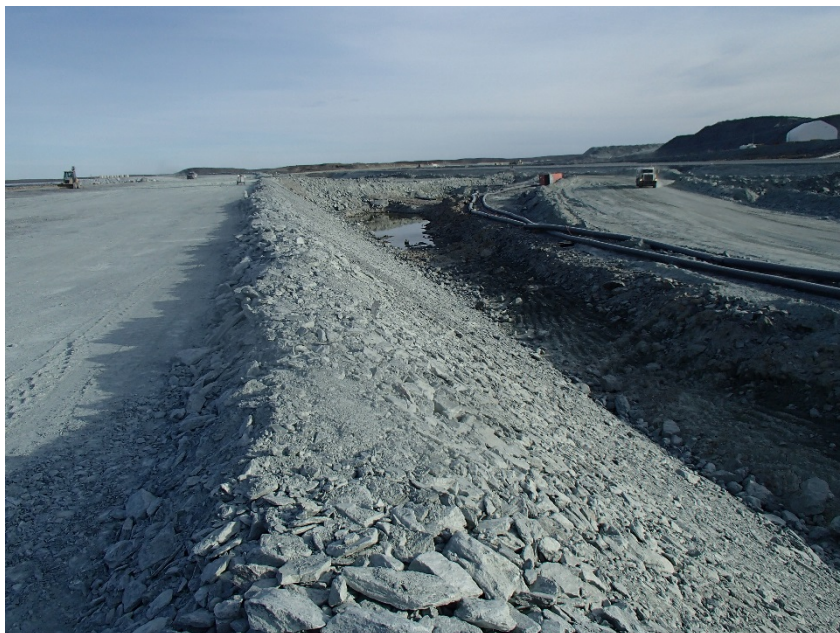
Photograph B6-6 Saddle Dam 4
