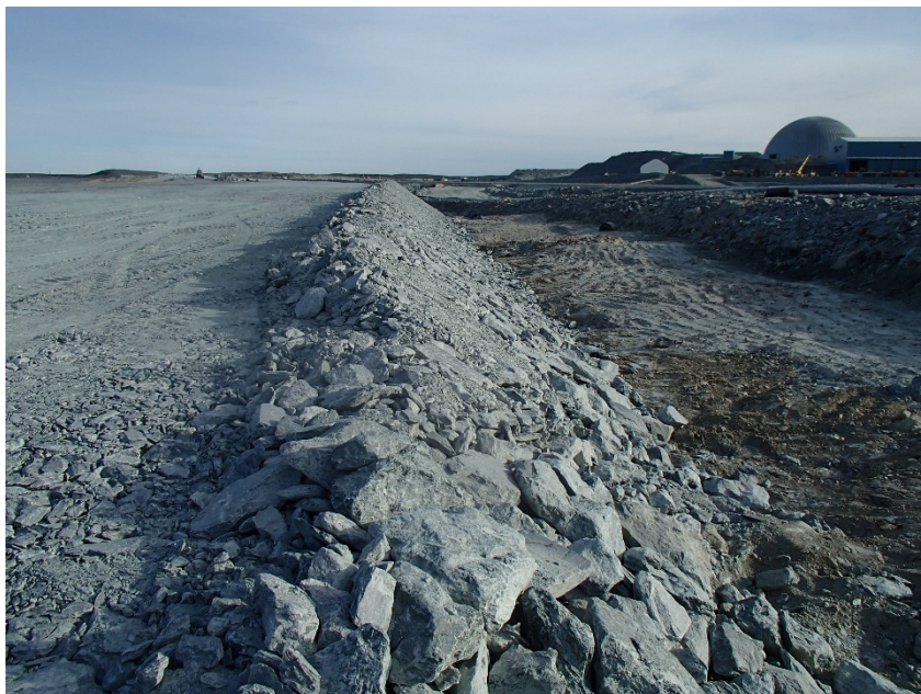
Photograph B6-2 Saddle Dam 4
