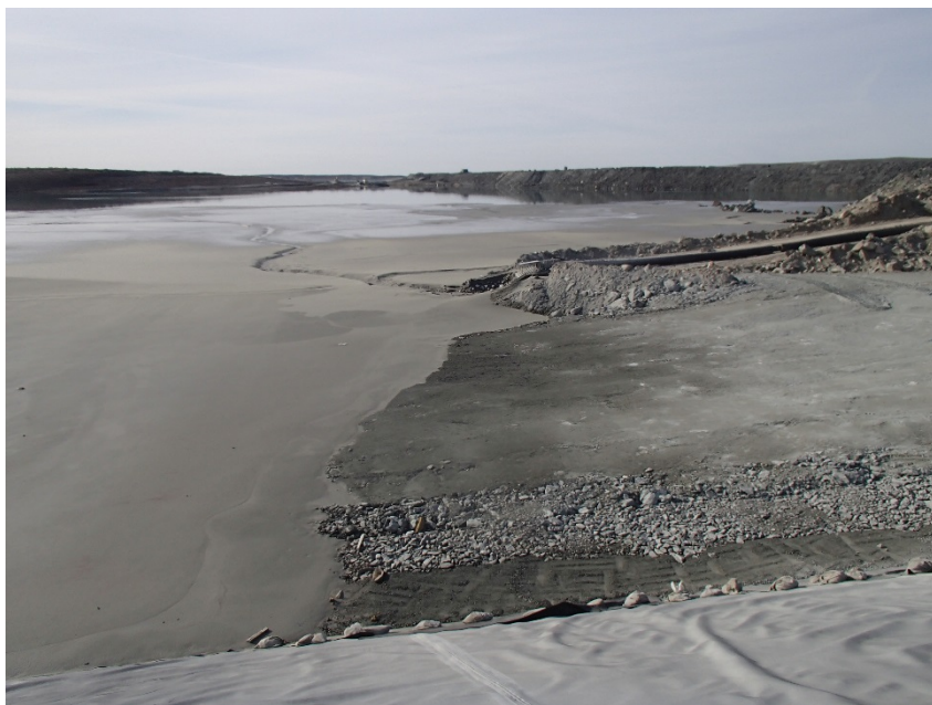
Photograph B7-2 Central Dike and Saddle Dam 5
