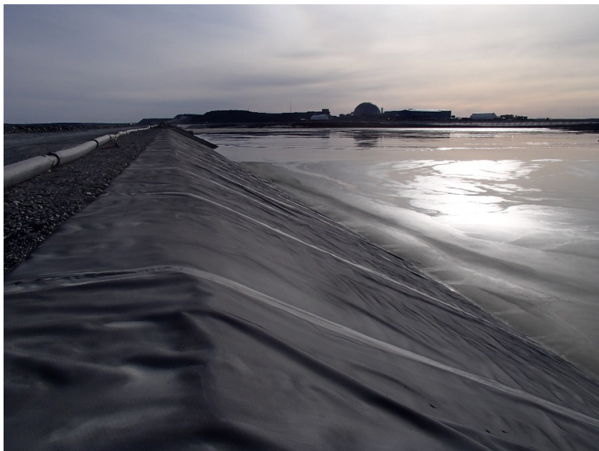
Photograph B7-1 Central Dike and Saddle Dam 5
