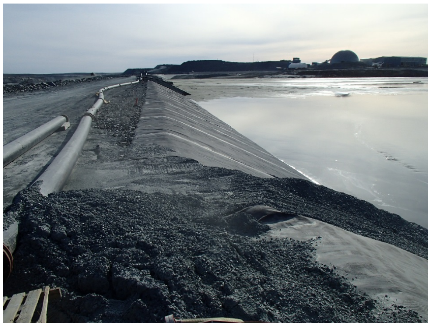
Photograph B7-6 Central Dike and Saddle Dam 5
