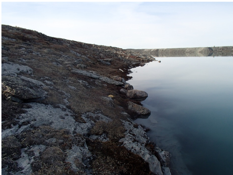
Photograph B6-9 Saddle Dam 4
