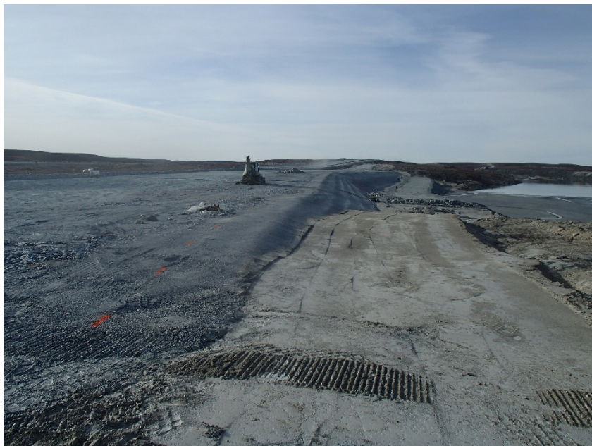
Photograph B6-1 Saddle Dam 4
