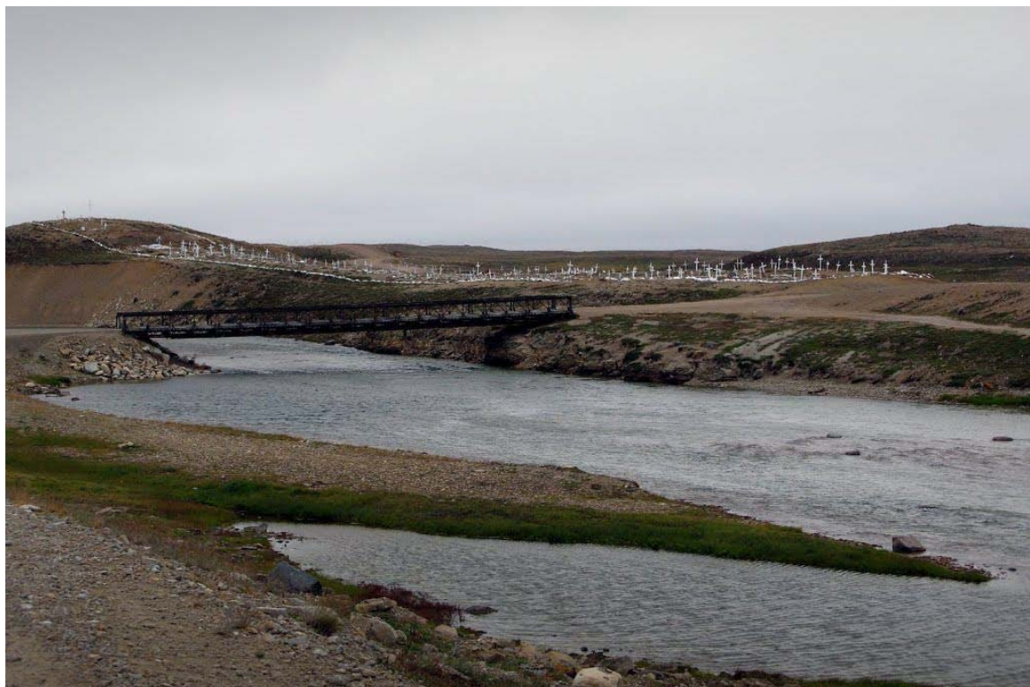
View of the Bridge at LWL in September
