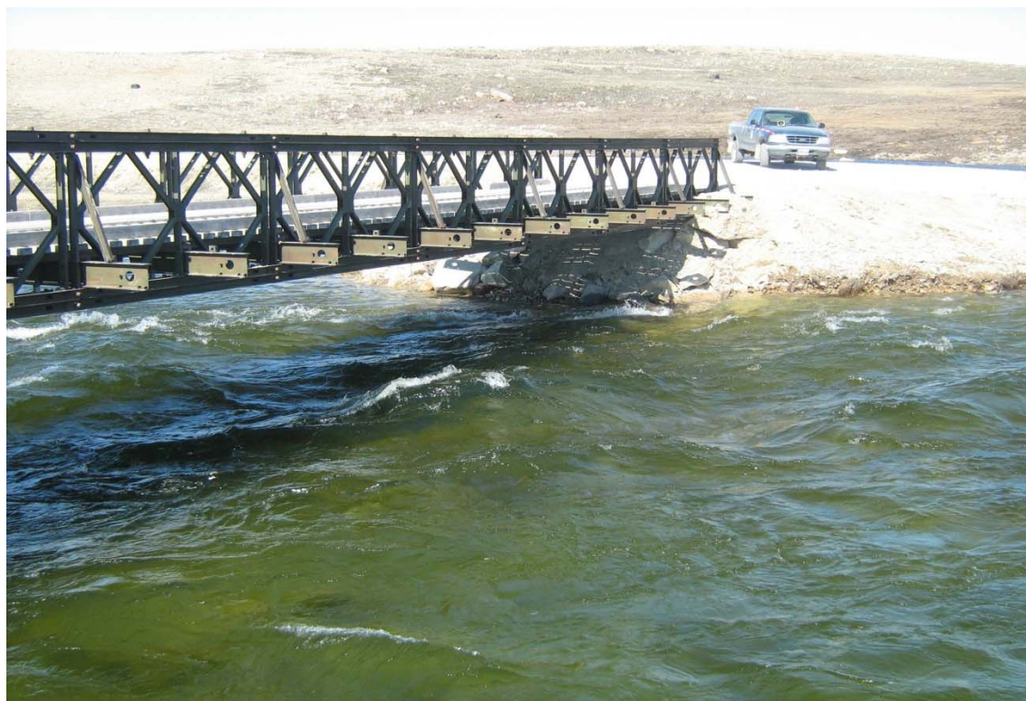
View of the Bridge at HWL in June
