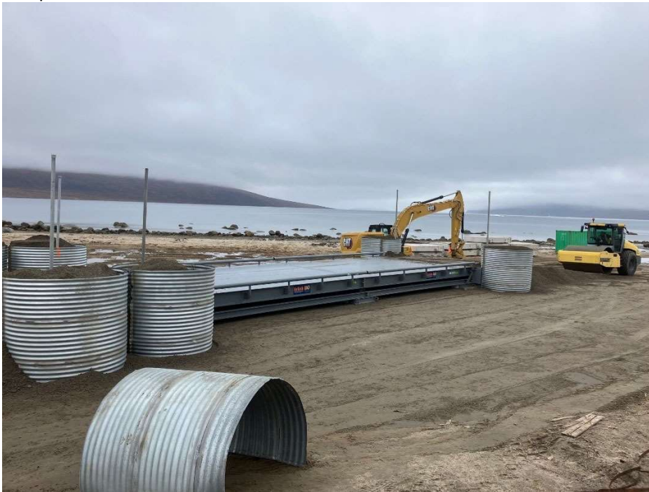
Weight scale installation
