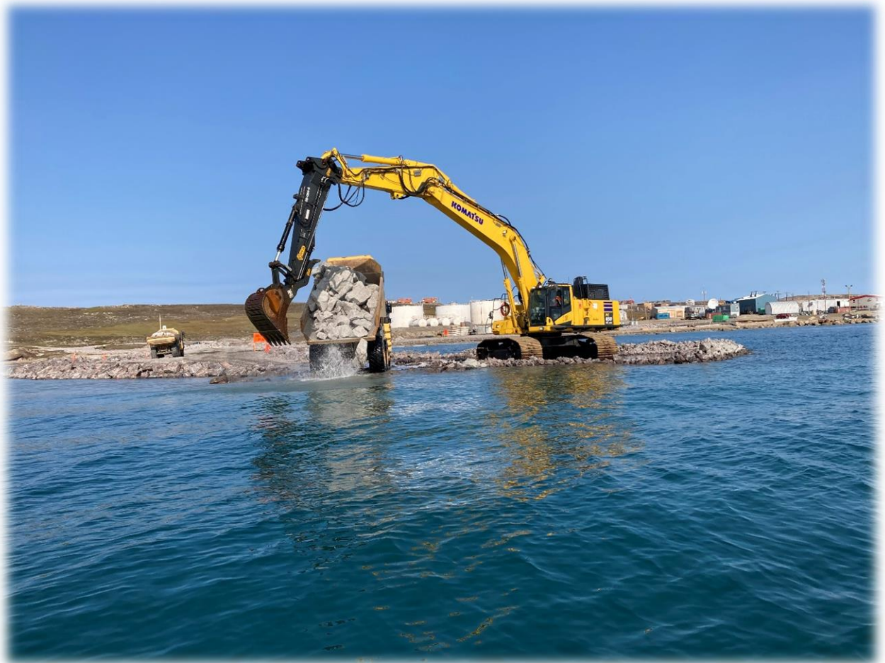
Southwest Breakwater Construction
