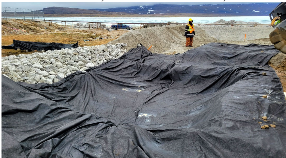
Picture 2.6.1: Construction of the sedimentation basin and the filtration berm
