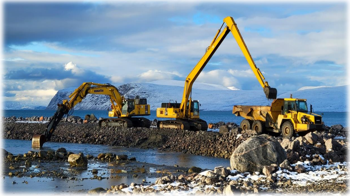
Dredging Along the Southwest Breakwater
