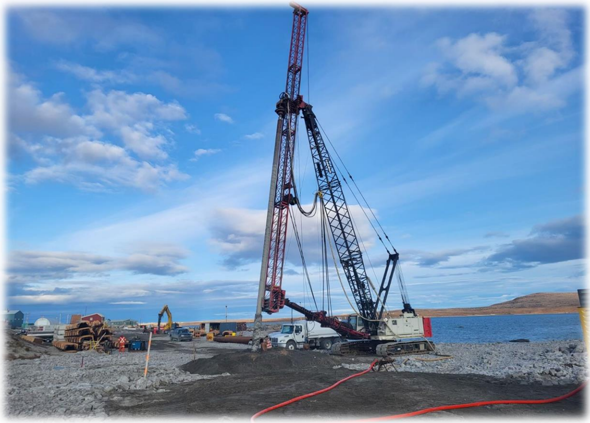
Drilling for the Mooring Bollard Installation
