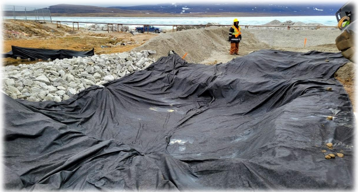
Dredge Spoil Storage Area Preparation
