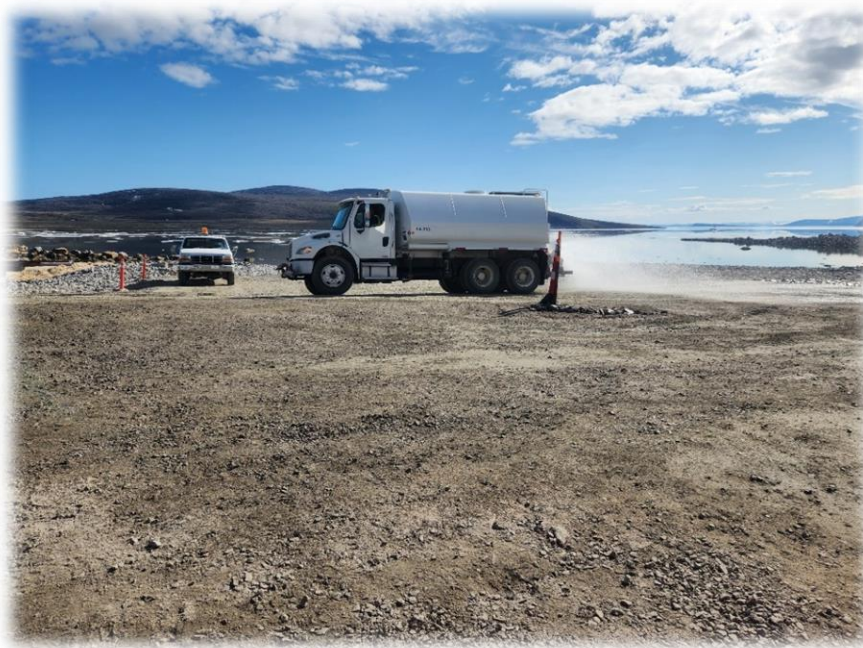
Water Spreading on the Road for Dust Control
