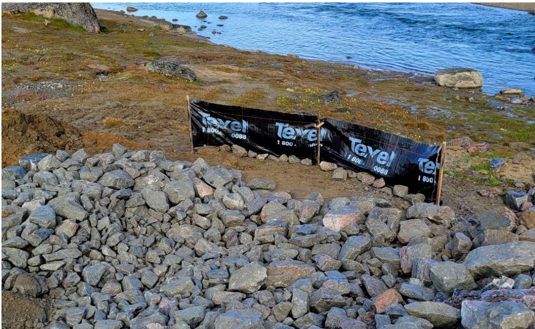
Picture 2.3.4: Catchment basin completed, silt fence was removed later
