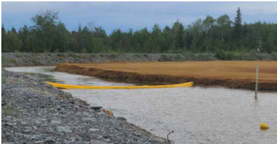
Typical installation of type 3 floating silt curtain
