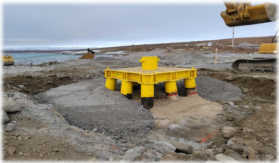
Mooring Bollard Installation Completed
