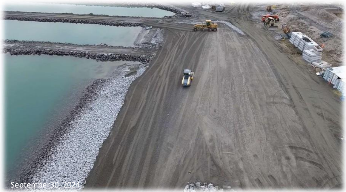
Uplands Upgrade -Crushed Stone Compaction
