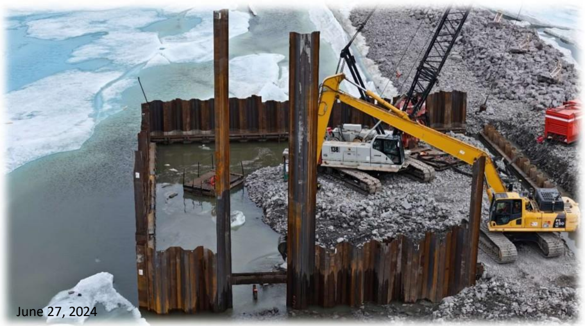
Fixed Wharf Construction: Sheet Piles Installation
