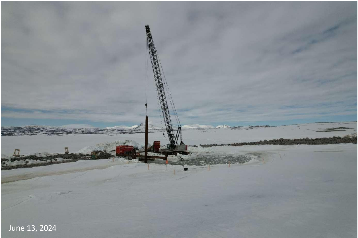
Fixed Wharf Construction: First Sheet Piles Installation
