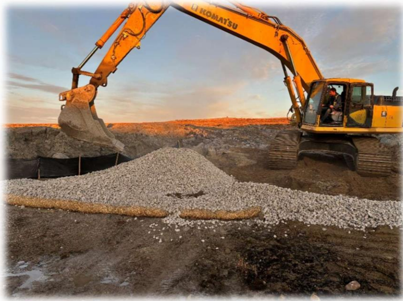
Filtration Berm Built at the North Corner of the of the DSDA
