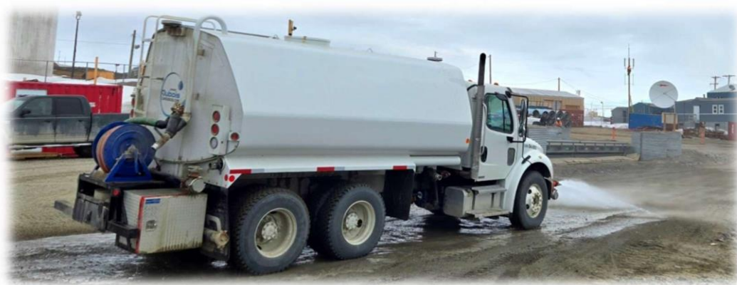
Water Spreading on the Road for Dust Control
