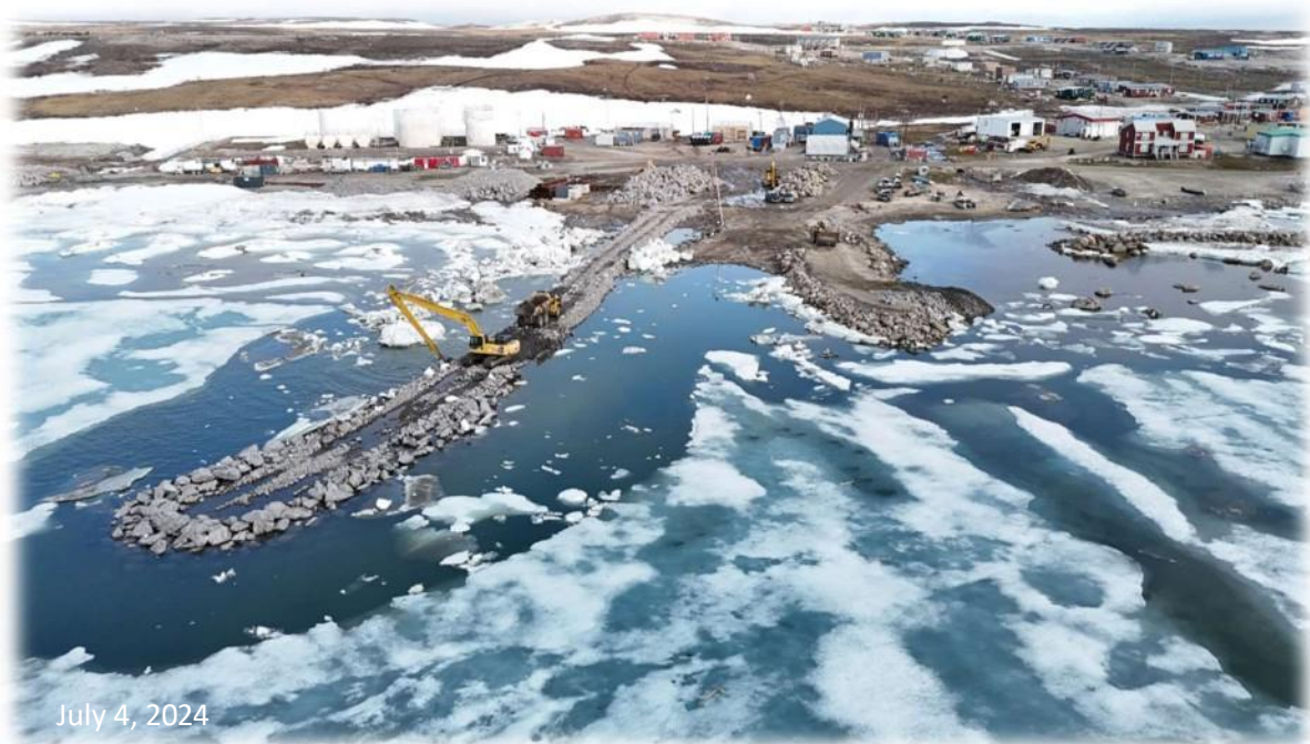
Northeast Breakwater Construction Beside the Existing Sealift Breakwater
