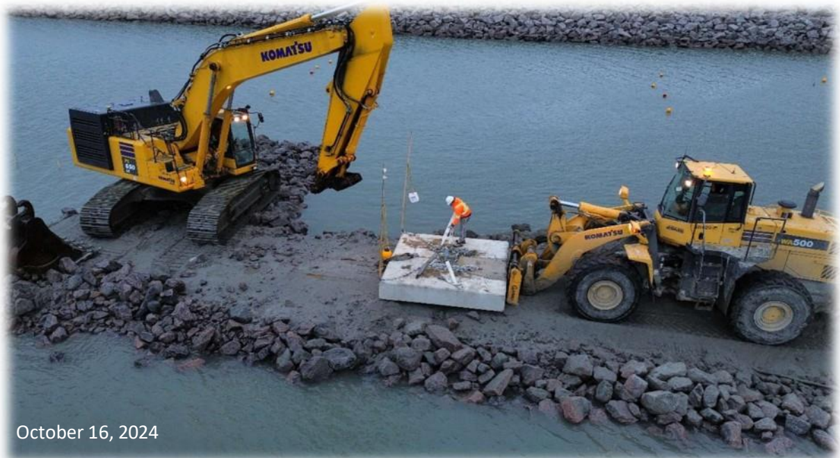
Installation of one of the 56 Concrete Anchor Blocks for the Floating Wharfs
