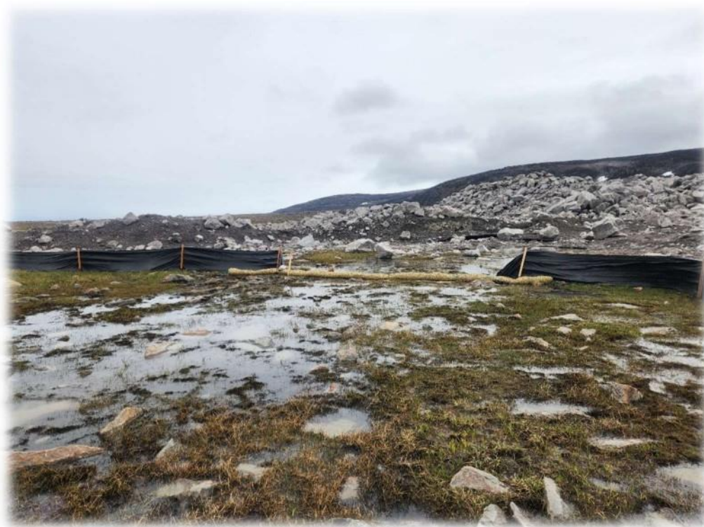
Silt Fences and Hay Logs Installed Between the Wetland and the Quarry North End
