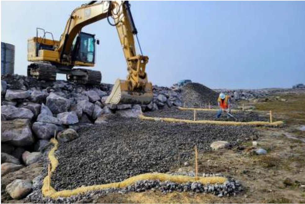
Picture 2.3.1 Erosion and sedimentation protection -Northeast side of Bridge
