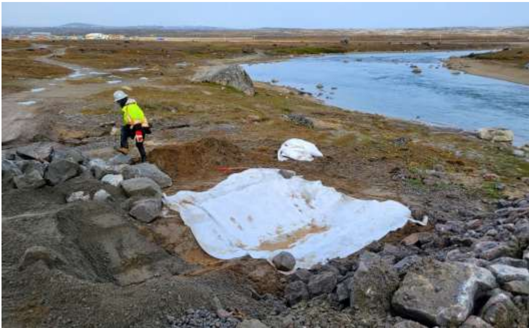
Picture 2.3.3: Catchment basin construction south side of the bridge
