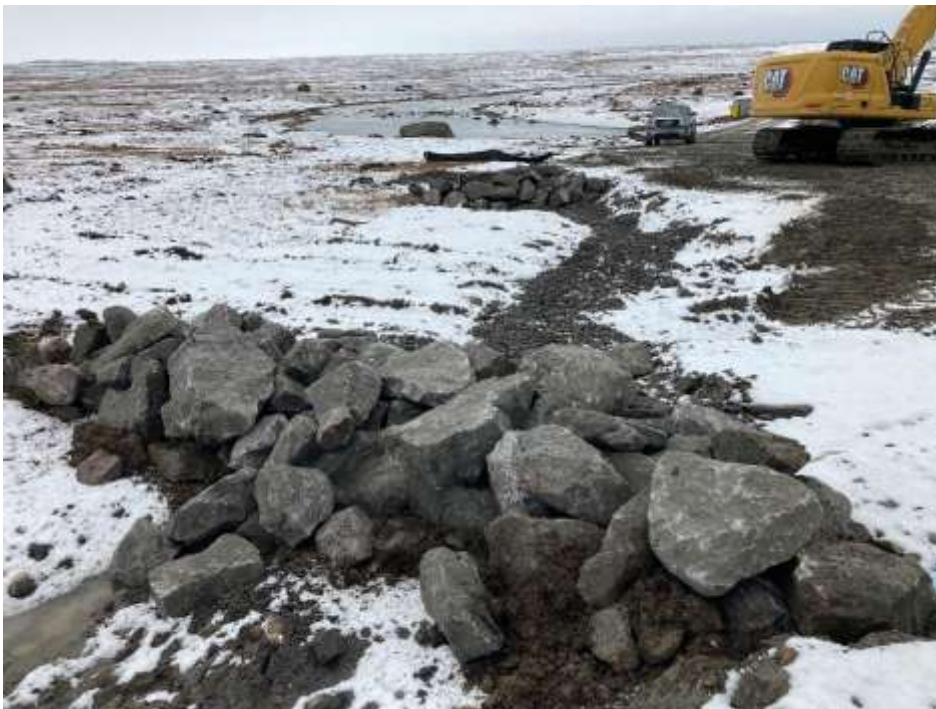
Picture 2.3.2: Checker dams built along the southwest side of the bridge approach
