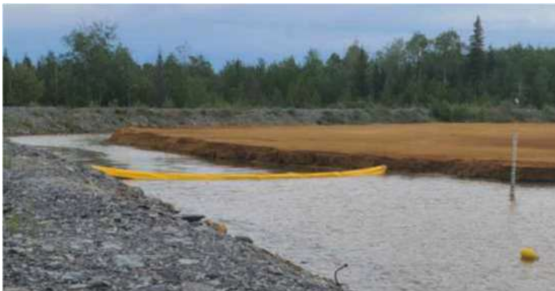
Typical installation of type 3 floating silt curtain
