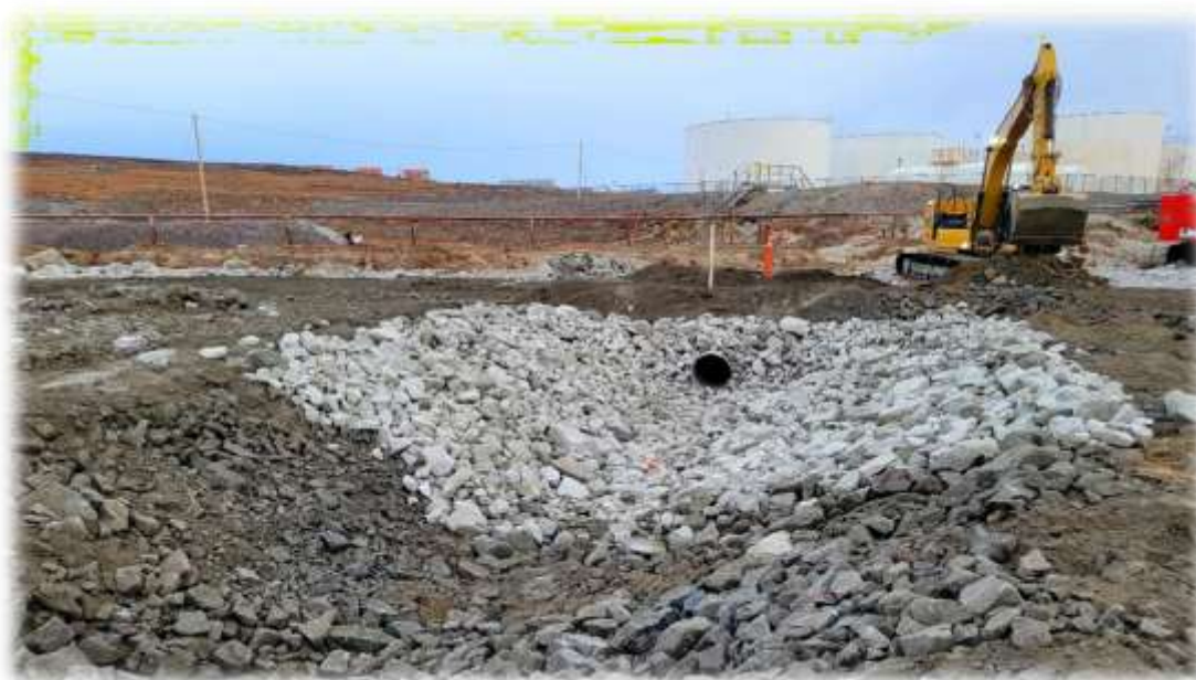
New Culvert and Erosion Protection Installed Under Access Road to Dewatering Area
