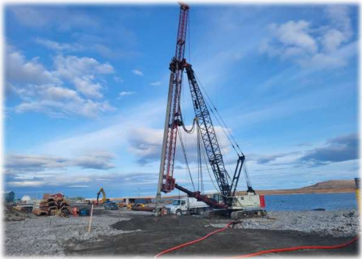
Drilling for the Mooring Bollard Installation
