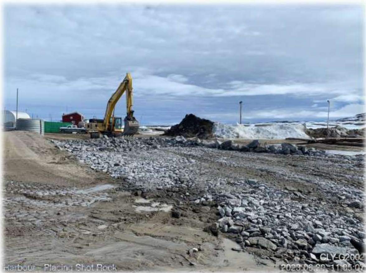
Placing Shot Rock on the Upland Area (in Front of the Harbour)
