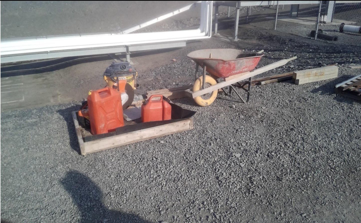
Description:2 x fuel tanks in secondary containment.
