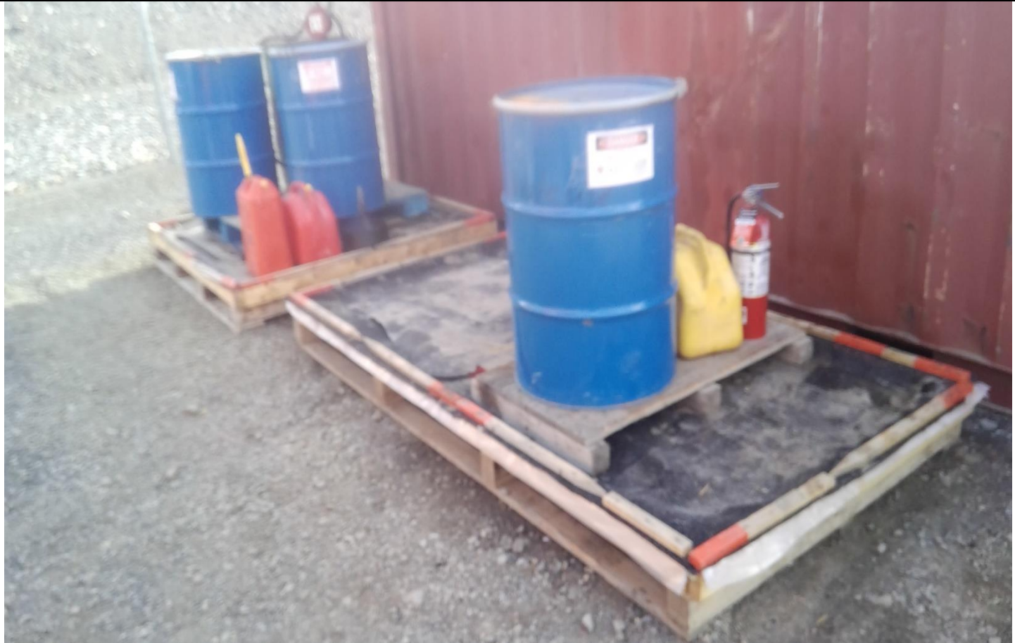
Description: Hazardous material placement, in secondary containment. Fuel pump, and ope
