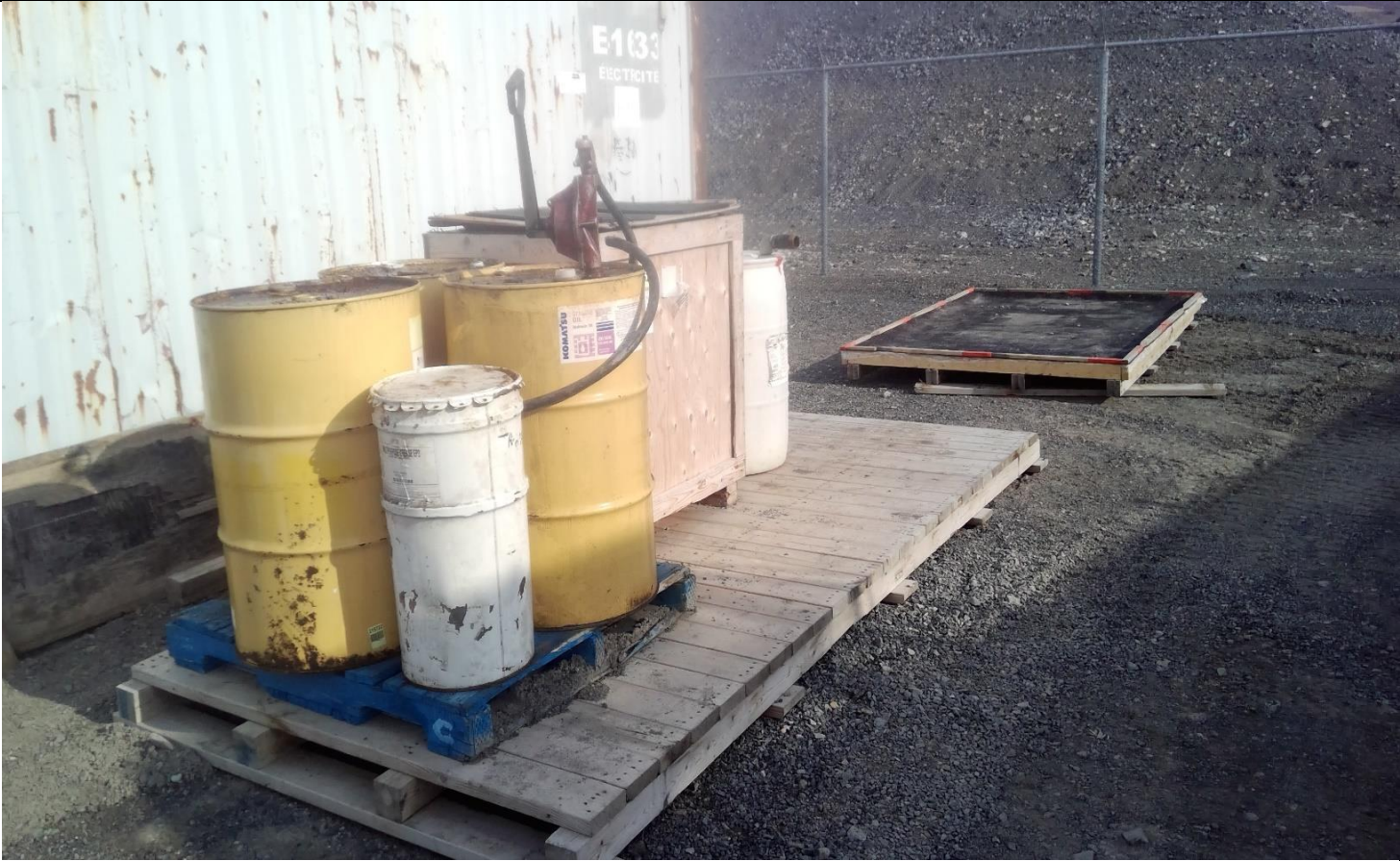
Description: Fuel Transfer Station. No secondary containment. No signs of spills.
