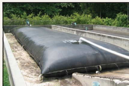
Geotube® unit in municipal wastewater treatment drying beds.
