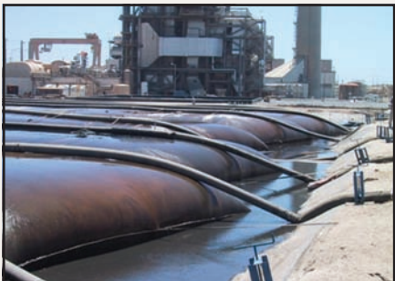
Geotube® containers at fossil fuel power plant being used to dewater fly ash.
