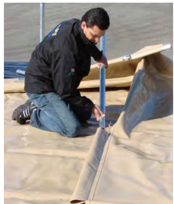
Sliding rails on a 20" high berm.
