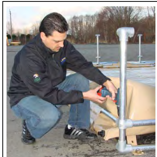
Lower rails in place and tighten set screw.
