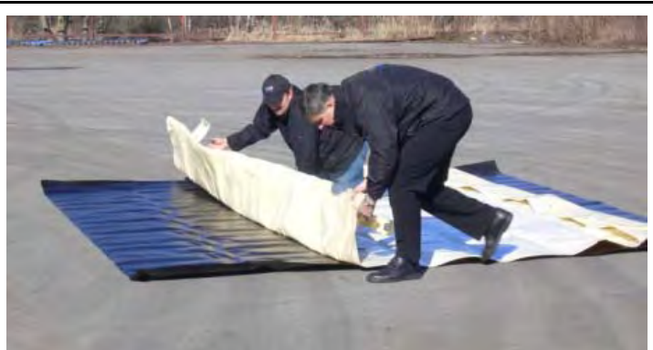
Folding the berm liner.
