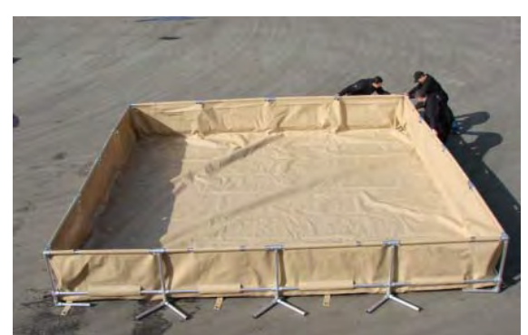
Attaching the top rail to the side post.
