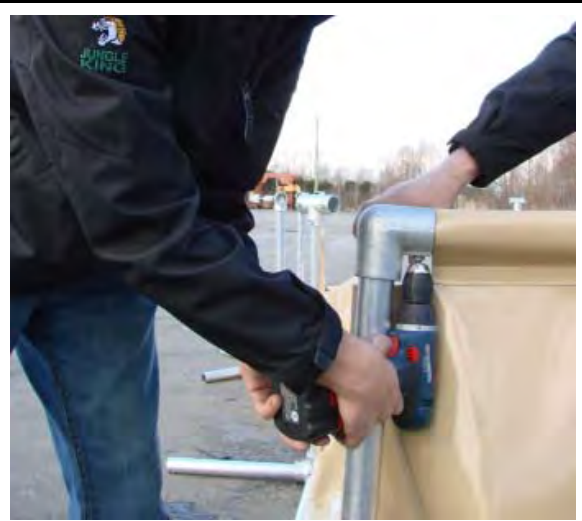
Tightening the top rail.
