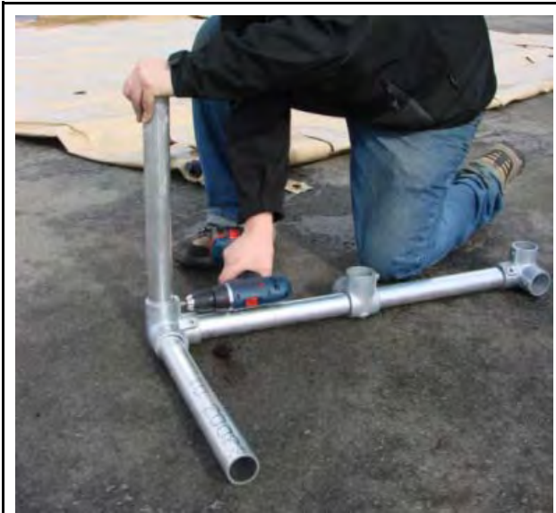
Tightening the leg set screws.
