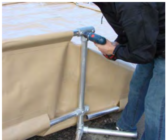
Attaching the top rail to the side post.
