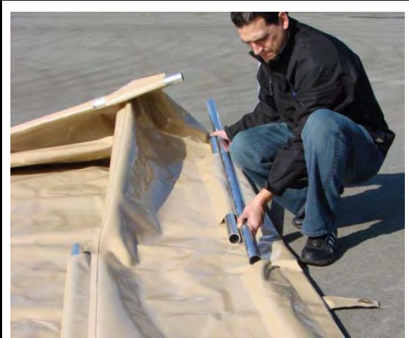
Slide top and bottom rails into pockets.
