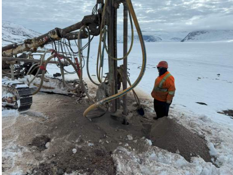
Photograph 5 Drilling an upland borehole.
