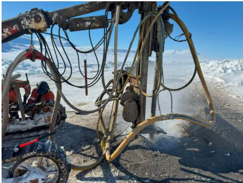
Photograph 4 Drilling an upland borehole.
