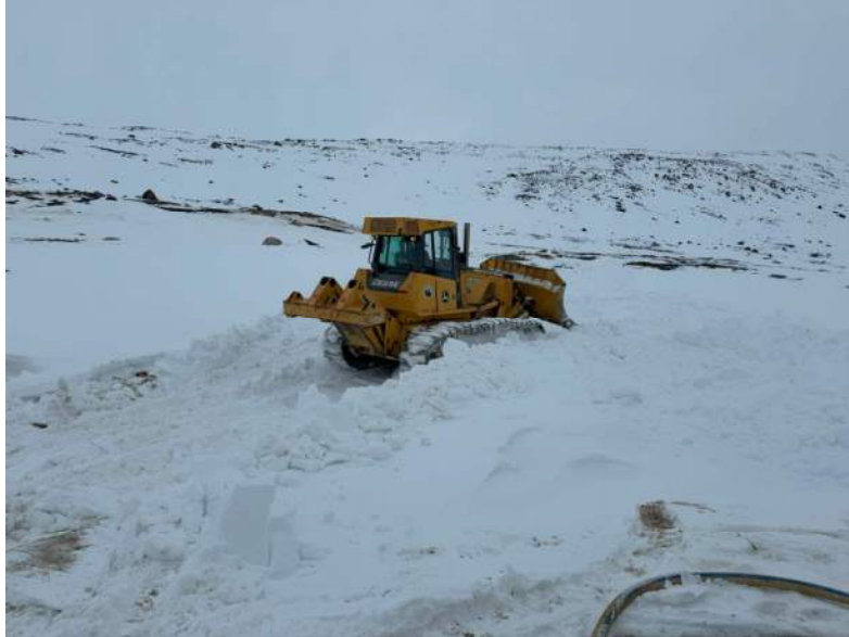
Photograph 3 Clearing snow for air-track drilling on the uplands.
