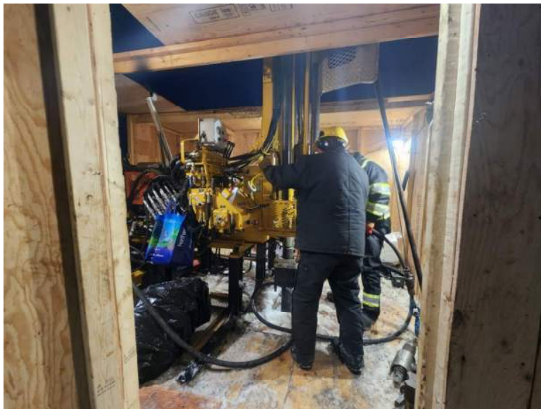
Photograph 12 Drilling a waterlot borehole.
