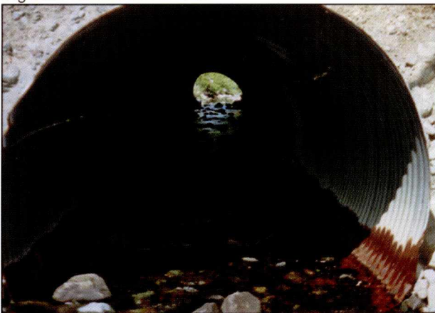
Figure 3. Countersunk Culvert
