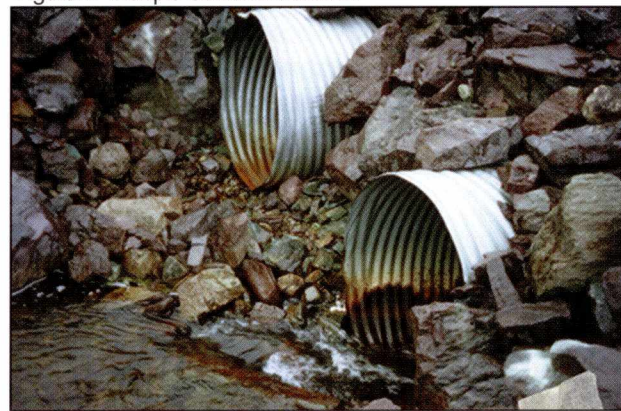
Figure 4. Multiple Culvert Installation
