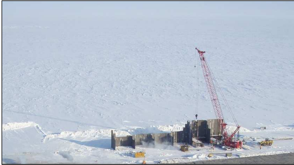
Plate 1.7-3. Causeway and wharf under construction in winter, Beaufort Sea.
