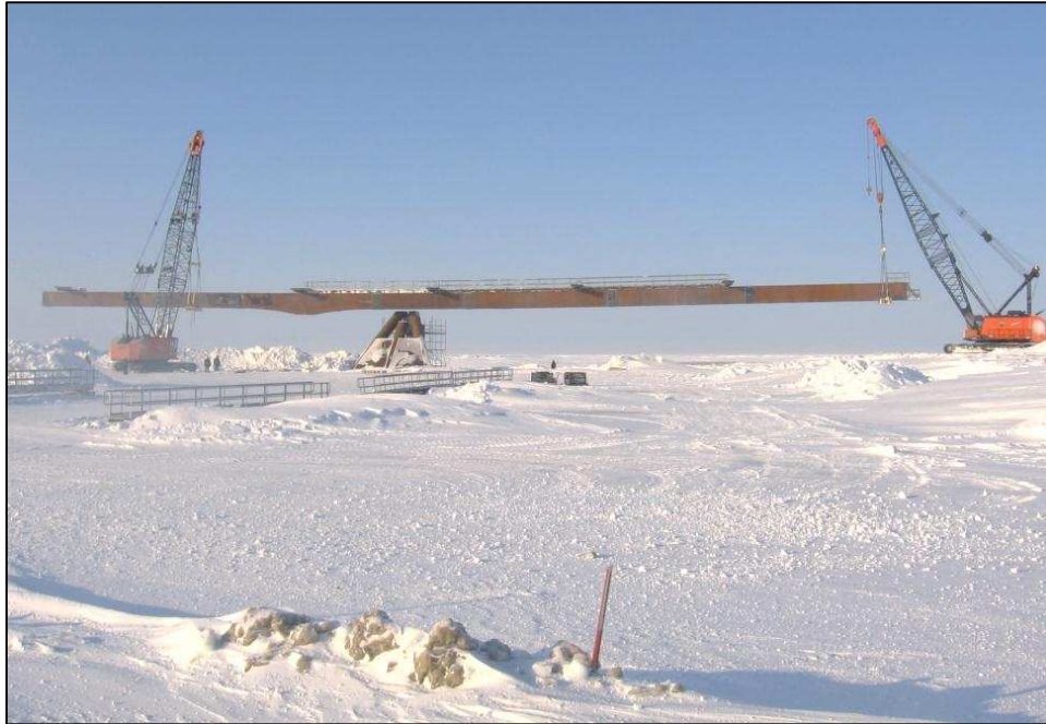
Plate 1.7-2. Lifting bridge girder sections from grounded ice, Kuparuk River, Alaska.
