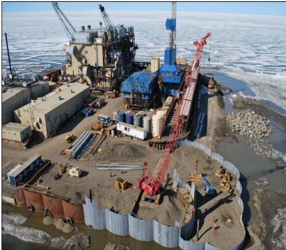
Plate 1.9-2. OPEN CELL reinforced earth bulkhead, Arctic Beaufort Sea.
