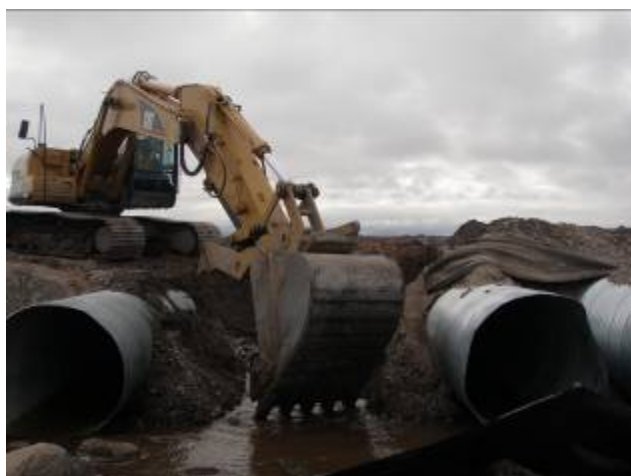
Figure 33 : Grading the Streambed
