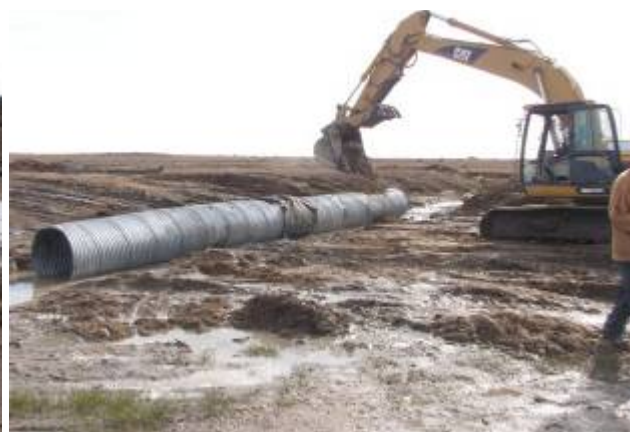
Figure 16 : Culvert Installation
