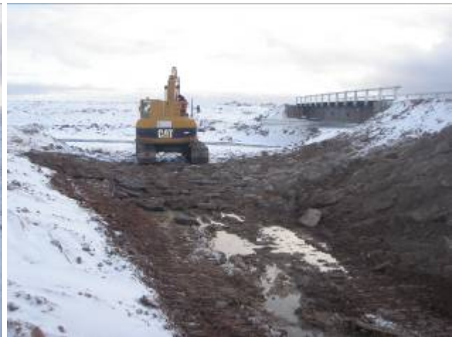
Figure 39 : Excavation of the Watercourse Figure 40: Opening to the River Closed
