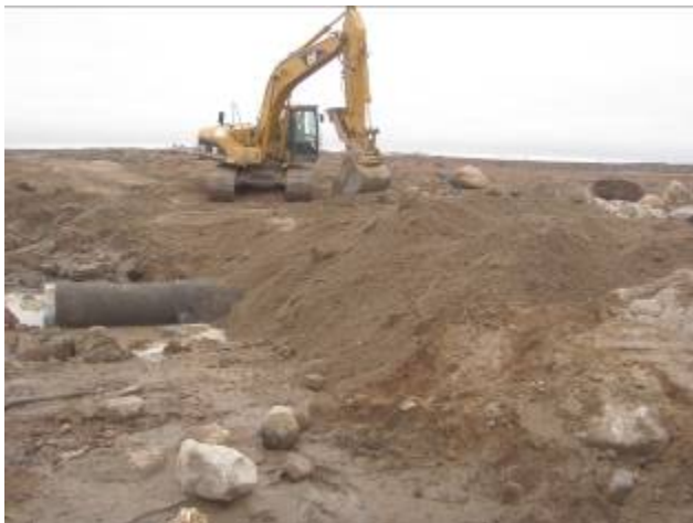
Figure 23 : Placement of Soil Cover
