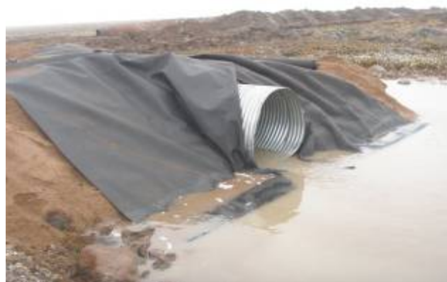
Figure 5 : Geotextile Placement
