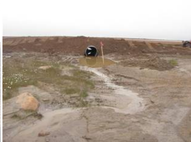
Figure 18 : Crossing 5 without Silt Fence
