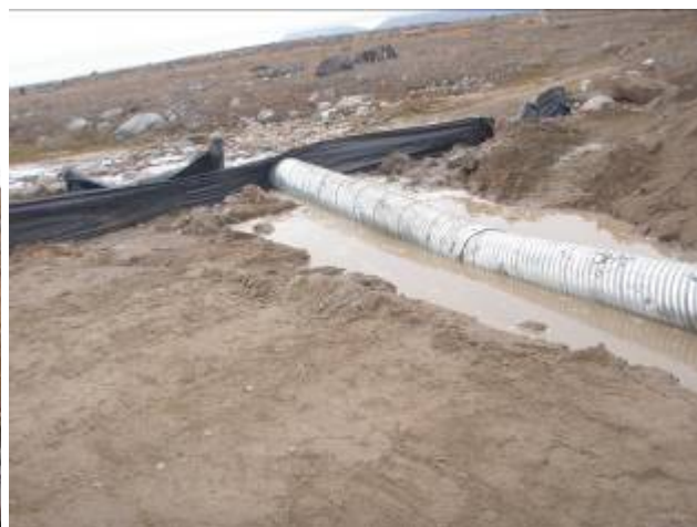
Figure 26 : Realignment of 36" Culvert
