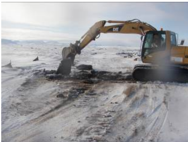
Figure 43 : Removal of Silt Fences
