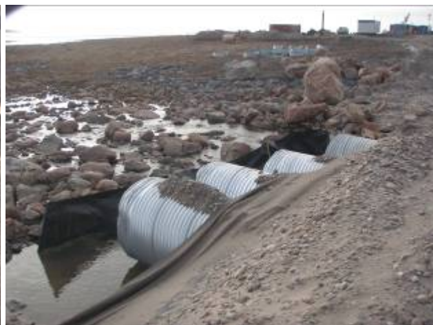
Fig 32: Silt Fence prior to Culvert Removal
