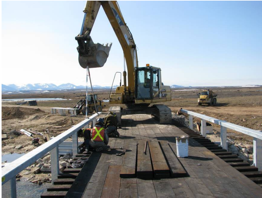
Figure 3: Installing the Bridge Rail
