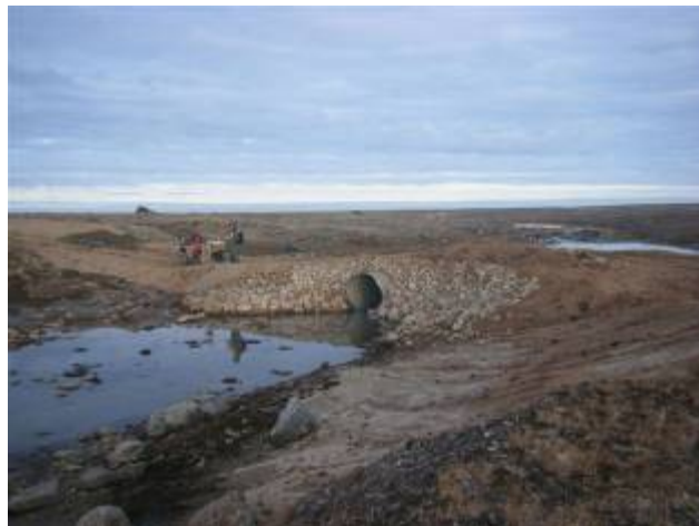
Figure 8 : Final Rip Rap Cover- North Side
