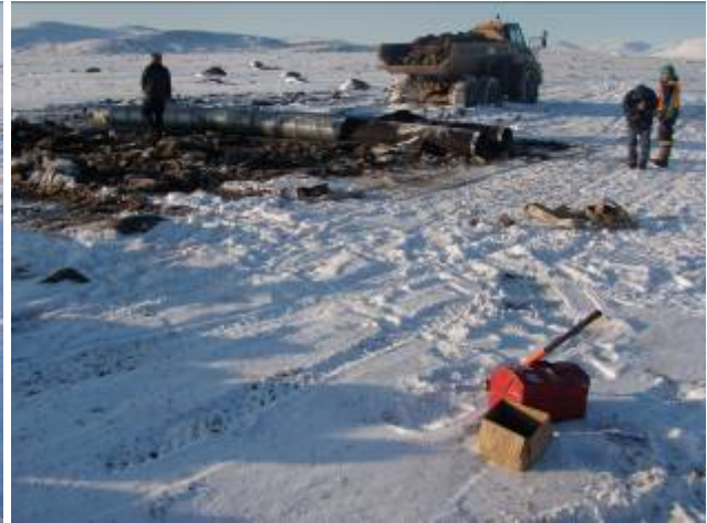
Figure 12 : Culvert Installation
