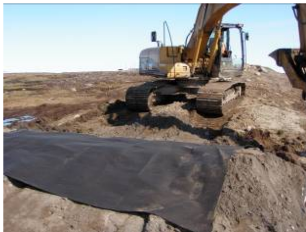
Figure 36 : Geotextile Placement
