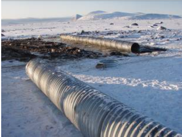
Figure 11 : Laying out the Culverts
