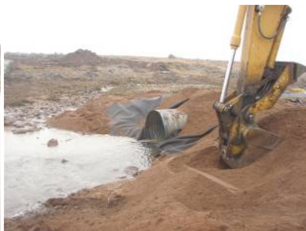
Figure 6 : Soil Placement
