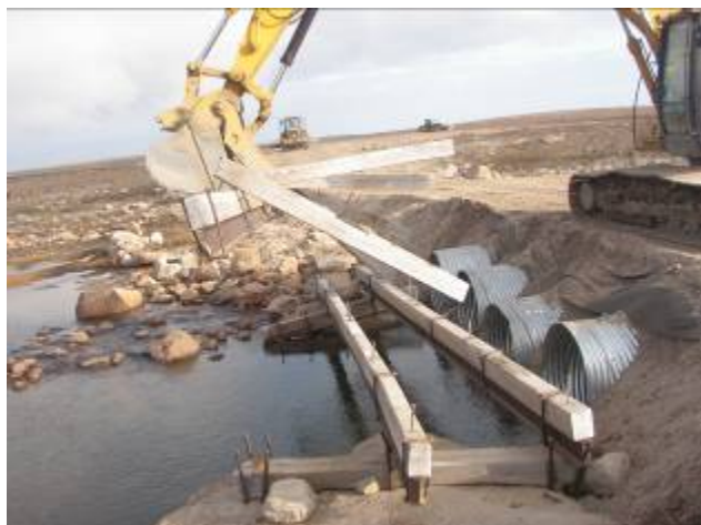
Figure 31 : Wooden Bridge Removal
