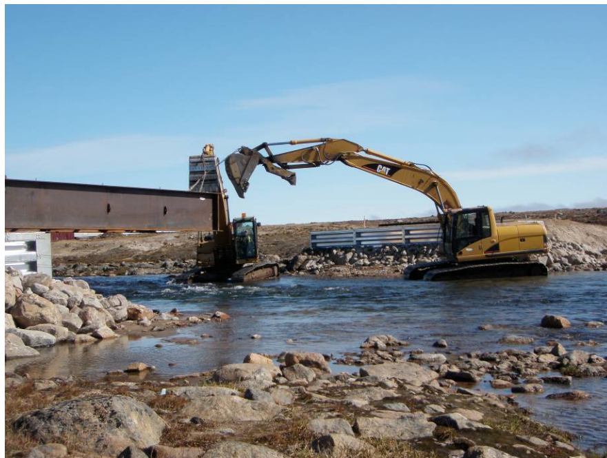
Figure 2: Pulling the Bridge Superstructure into Place
