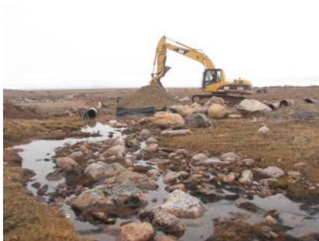
Figure 25 : Removal of Soil Cover
