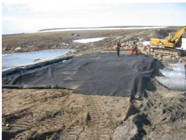
Figure 29 : Geotextile Placement
