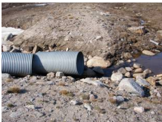
Figure 37 : Laying out the Culvert
