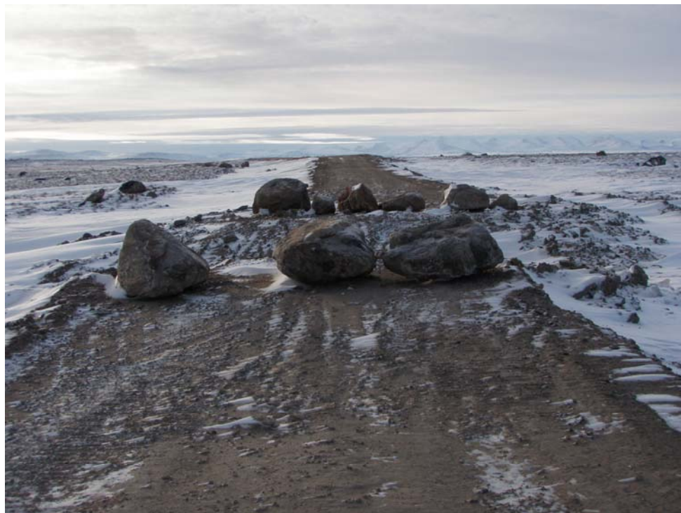
Figure 5 : crossing 11 after removal of the culvert
