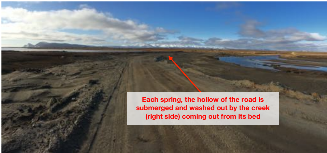
Photo 10: Stability issue near stream crossing #4, Km 4.7
