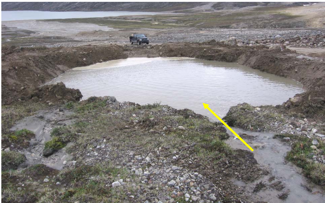
Figure 6 : Check Dam and Runoff Flow Direction (FOX-C 2006)
