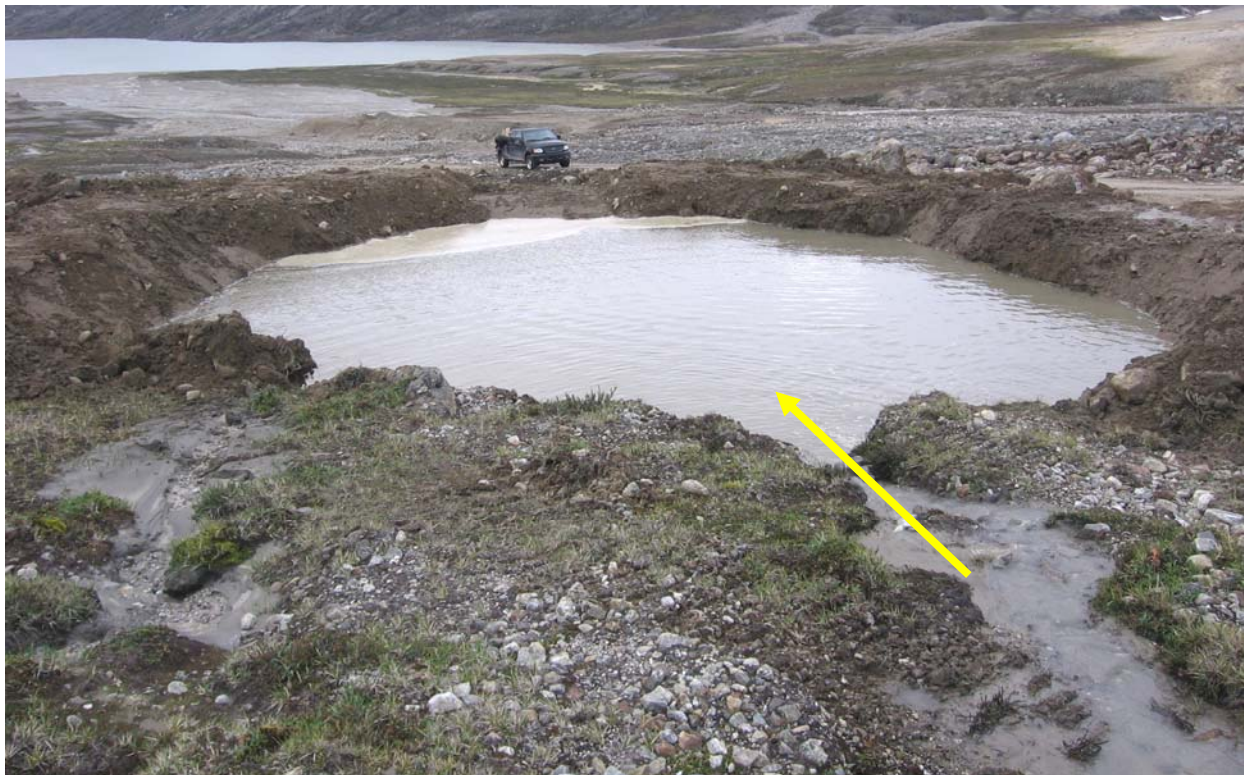
Figure 6 : Check Dam and Runoff Flow Direction (FOX-C 2006)
