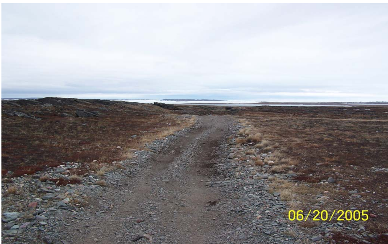
Photo 2- Trail Section located on dry granular soils
