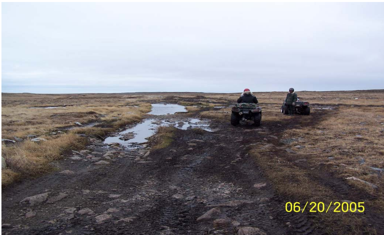
Photo 5 – Trail through fine grained soils, some embedded rocks and standing water
