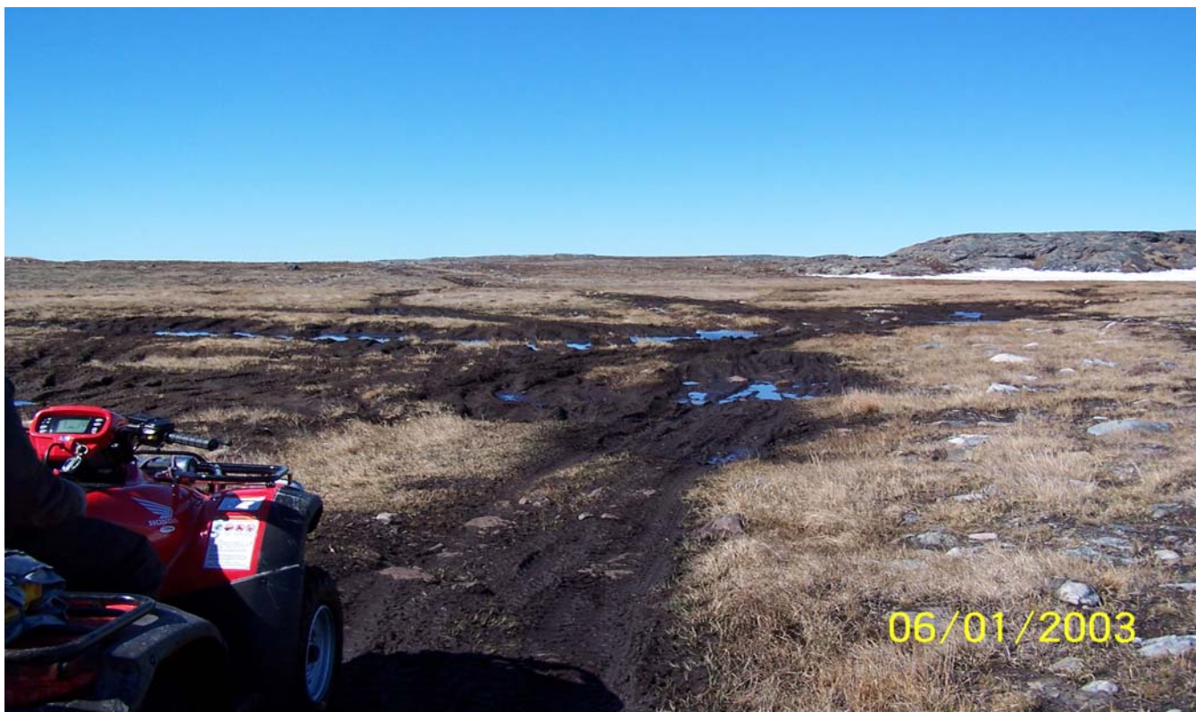
Photo 6 – Wet area in fine grained soils. Note trail widening.
