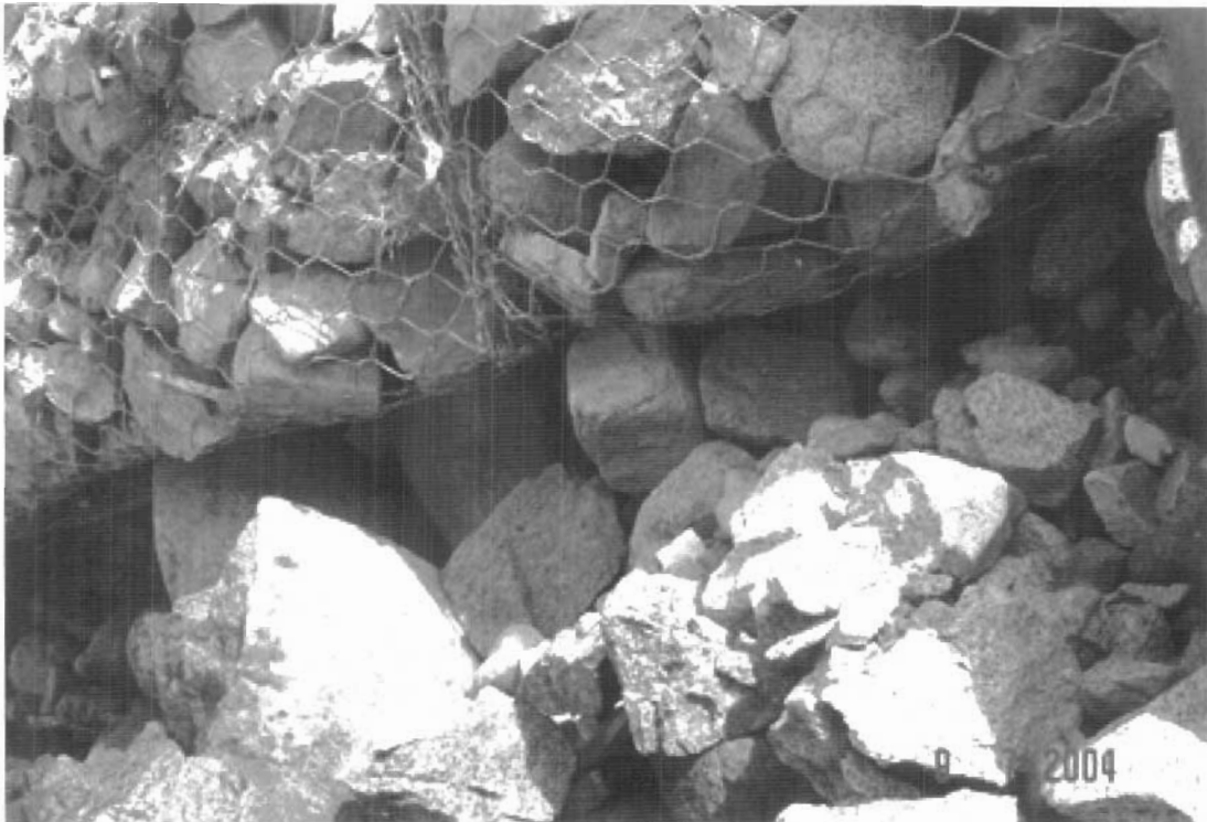
Base of gabions on east abutment. Boulders cracked and split under excessive weight
