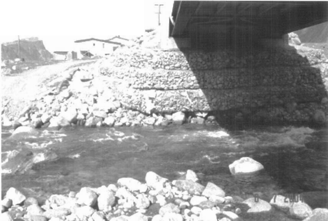
Head Slope of east abutment: 4.0 m section of gabion base is washed out. Gabions are point-supported on few larger boulders, some of which have cracked under the excessive load
