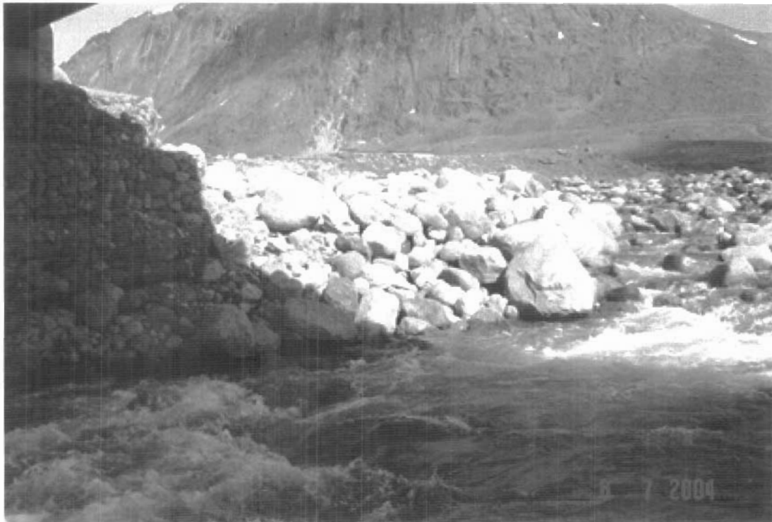
View of upstream part of east abutment. Rock berm placed on the upstream side and between abutments during repair around 1993. River current and ice traffic have washed out not less than one meter layer of rock
