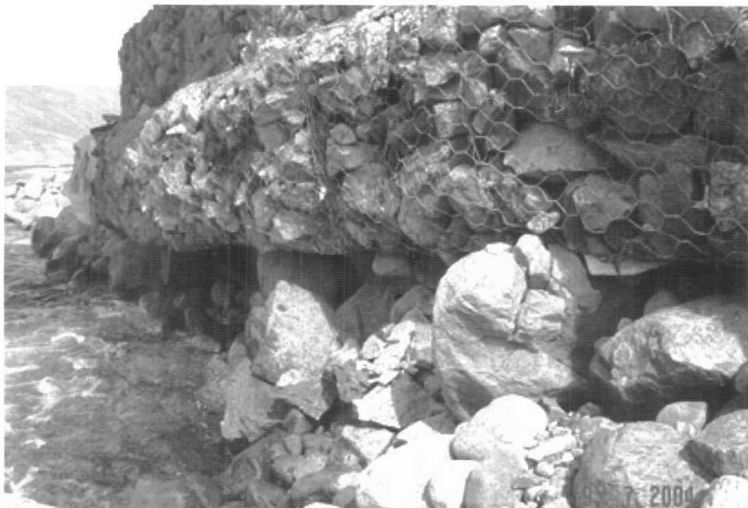
Gabions on east abutment. Boulder cracked under excessive weight (close plan to the right)
