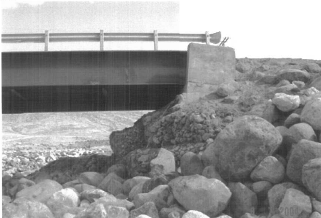
North elevation of west abutment: Evidence of "tilt" of abutment (pile cap); slump of gabions towards the river; and missing (washed out) gabions. Riverbed in front of gabions was washed out near 1992. Rock was placed in attempt to stabilise abutment.
