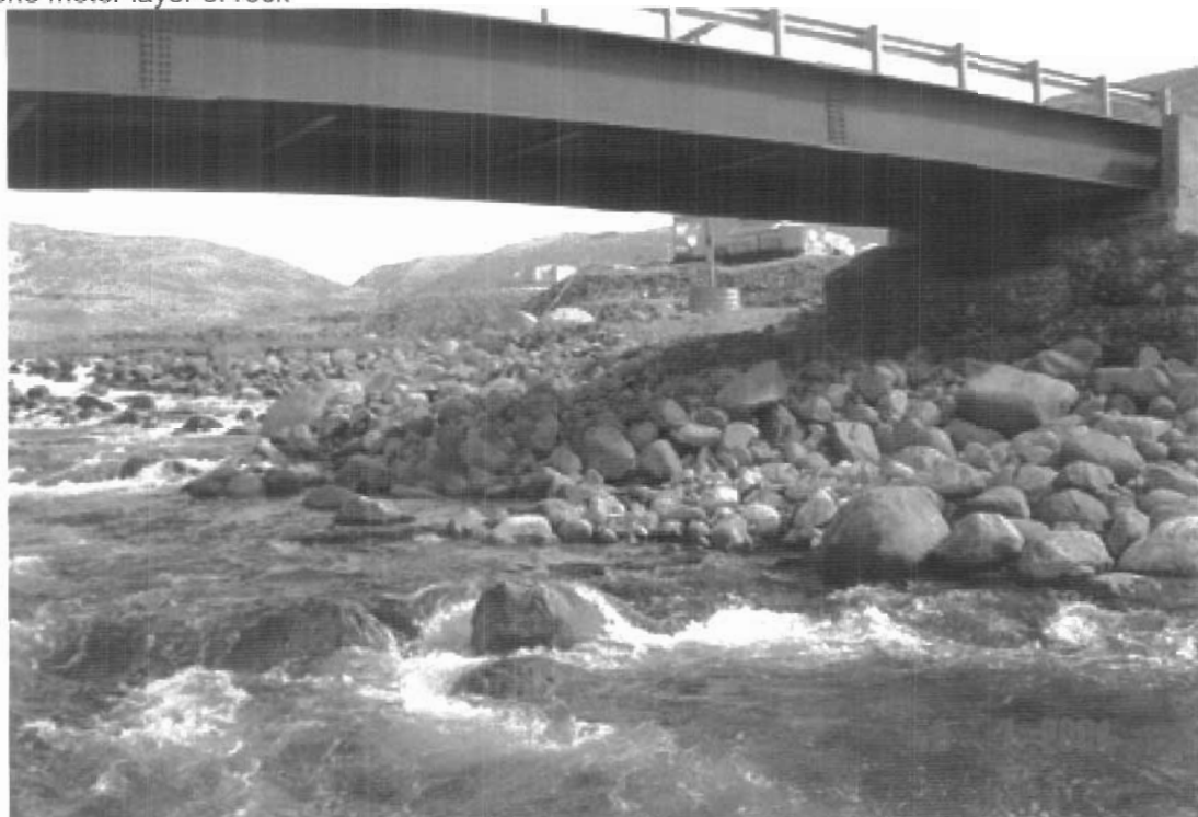
View of upstream part of west abutment. Rock berm placed on the upstream side and between abutments during repair around 1993. River current and ice traffic have washed out not less than one meter layer of rock
