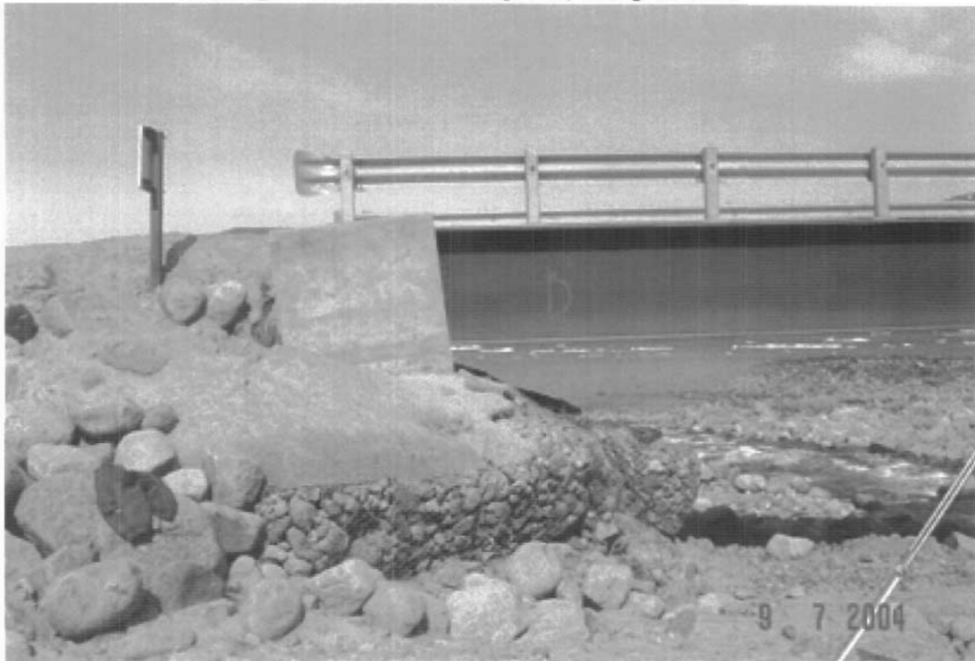
South elevation of west abutment: Evidence of "tilt" of the pile cap. Tilt is due to scour of riverbed under the pile cap; sliding of embankment towards the river; and failure (buckling) of steel piles supporting the cap. Pile cap is being held from sliding down by rebar tie-backs shown on pictures below
