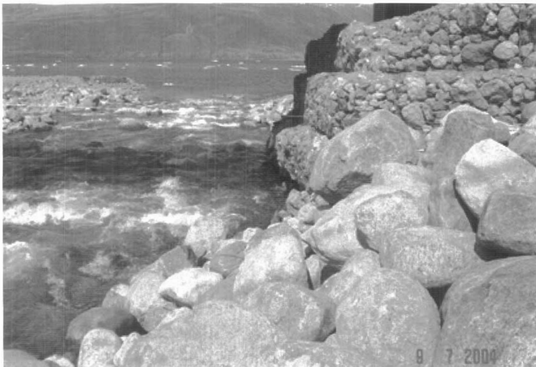
Current undermining the base of gabions on east abutment. In close plan: rock previously placed in attempt to protect abutment
