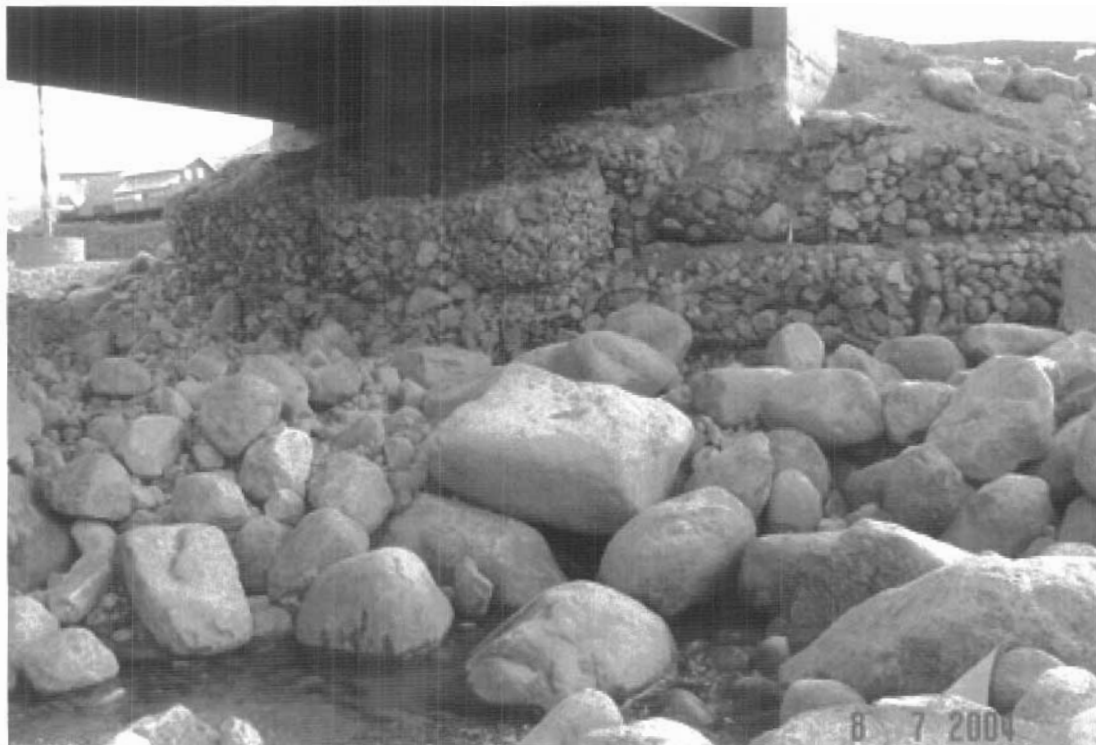
Head slope of west abutment: Riverbed in front of gabions was washed out near 1992. Rock was placed in attempt to stabilise abutment.
