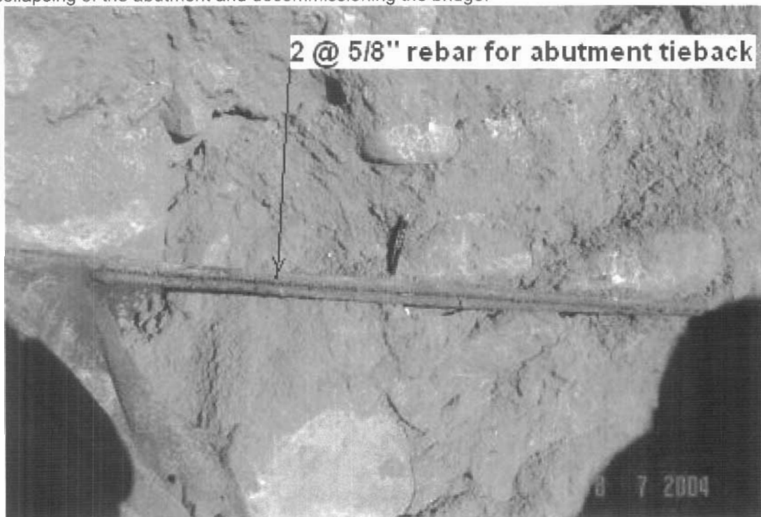
Detail of rebar tiebacks
