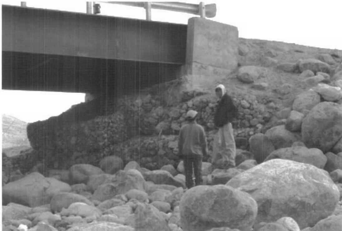
North elevation of west abutment: Evidence of "tilt" of abutment (pile cap); slump of gabions towards the river; and missing (washed out) gabions.
