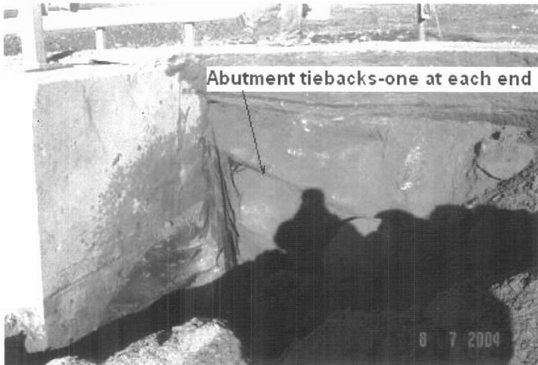
Excavation behind west (tilted) abutment. Note rebar tiebacks anchoring pile cap to dead man behind. Tiebacks are in good condition. Failure of these tiebacks will most certainly cause collapsing of the abutment and decommissioning the bridge.
