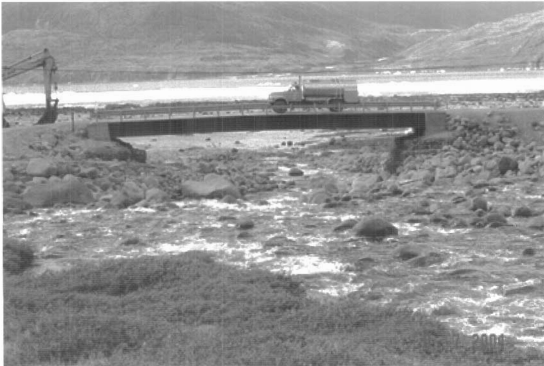
South Elevation of bridge: Reportedly the riverbed was built up to the top of Rock Berms visible in front of both abutments. The rock was placed during previous attempts to stabilize the riverbed.
