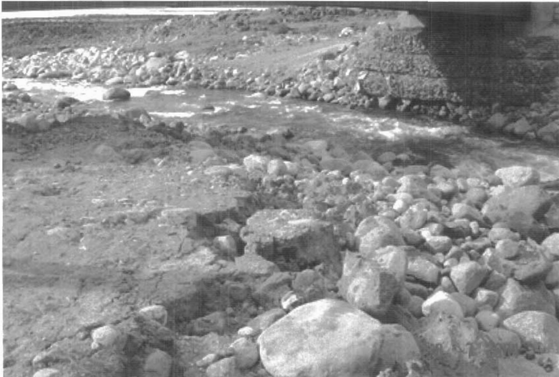
View of upstream side of west abutment. Evidence of failure (cracking and down-sliding) of the embankment due to undermining
